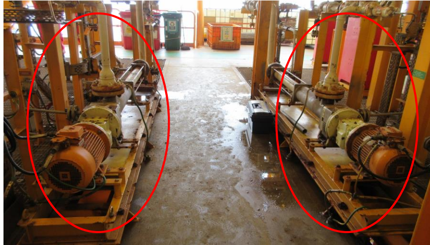
Condensate Booster Pumps (P-3401 A&B)
