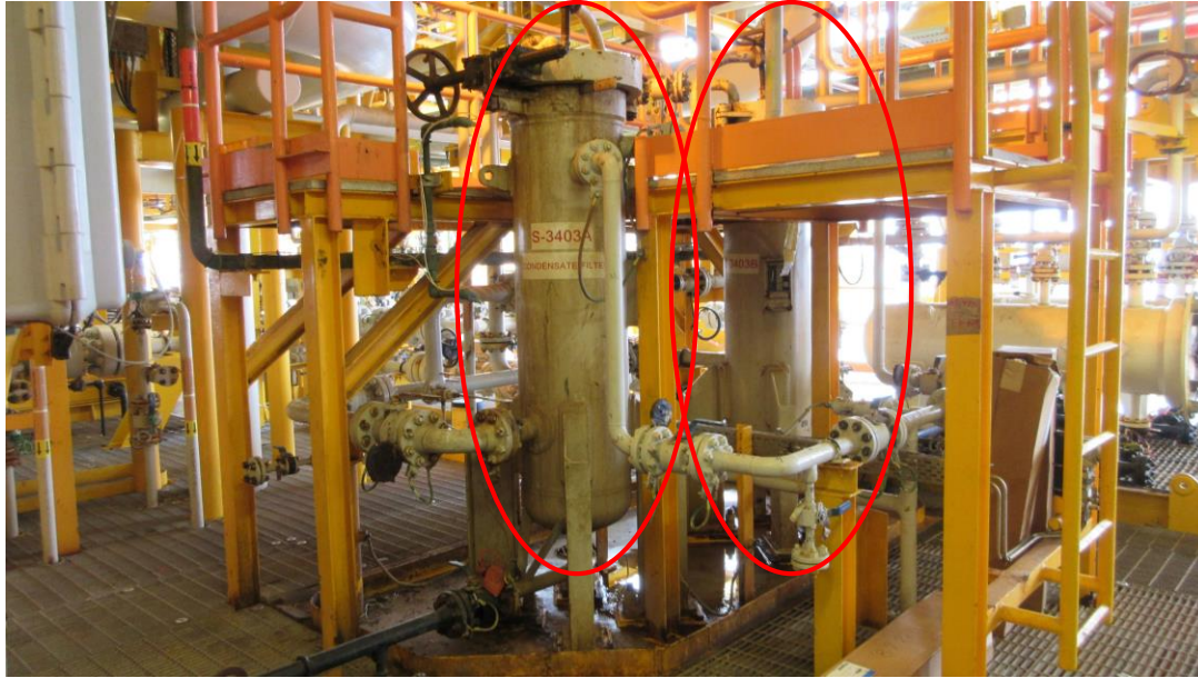
Condensate Filters (S-3403 A&B)
