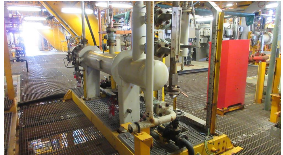
Produced Water Pre-Filter & Filter Coalescer Package (A-3703)
