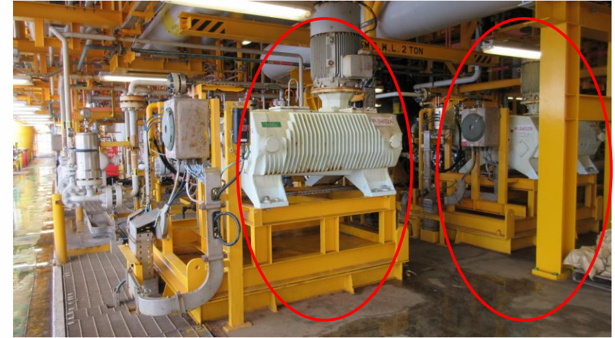
Liquid Re-injection Pumps (P-3402 A&B)
