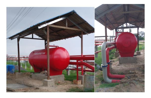
Figure: Fluroprotein Foam Storage Tank
