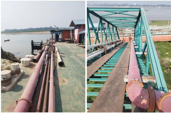
Figure: Pumped water system form Ayeyarwaddy River
