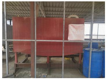
Figure: Diesel Storage Tanks for generator
