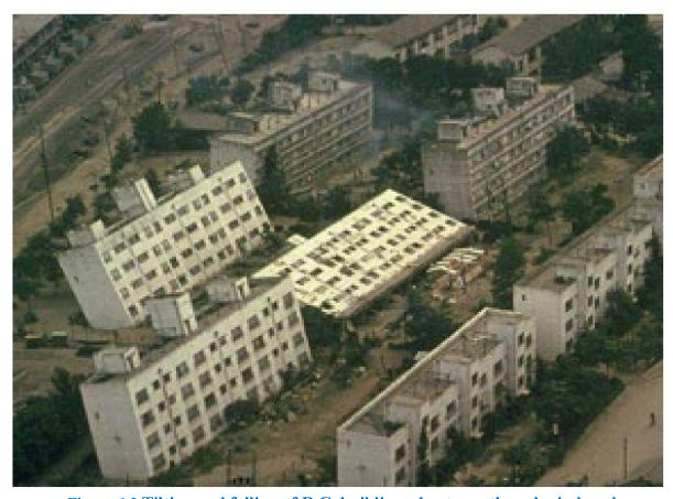
Figure 6.3 Tilting and falling of R.C. buildings due to earthquake-induced
