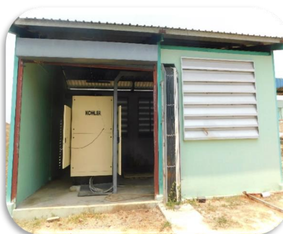
Transformer 11/0.4KV 500KVA and 350 KVA generator
