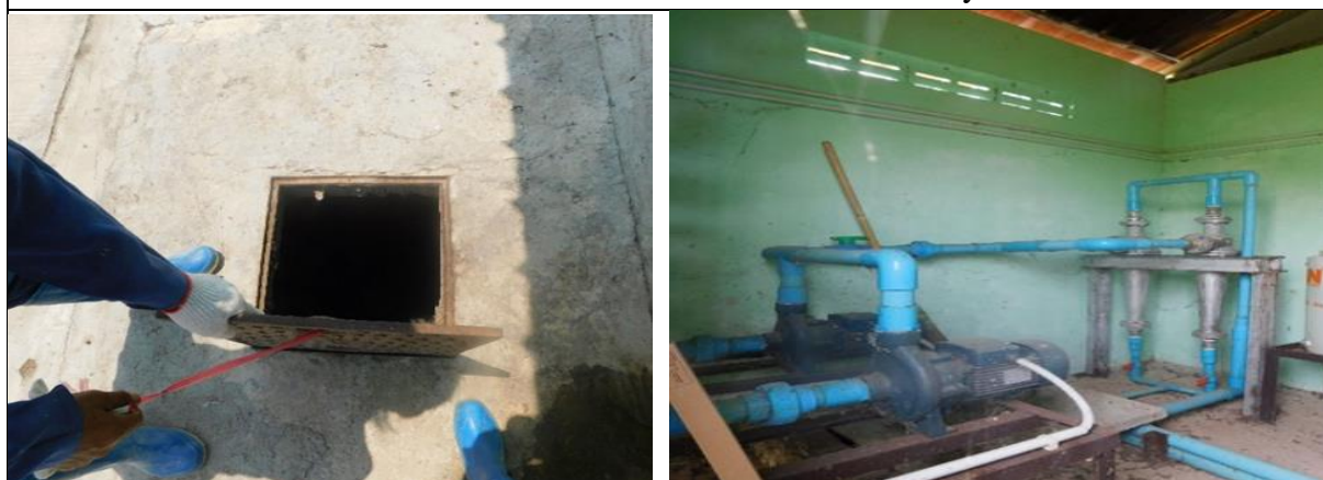
Wastewater collecting Tank and Pumping station at treatment facility
