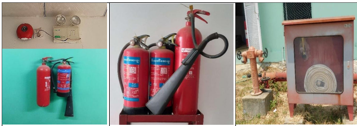
Figure 27. Fire extinguishers, hose, alarm and emergency lighting in PS farm 1
