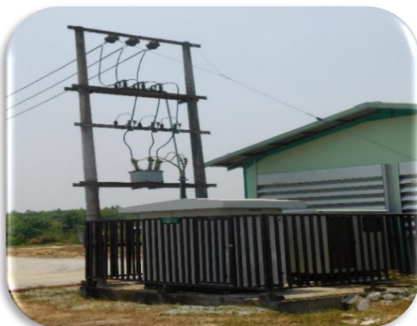
Transformer 11/0.4KV 500KVA and 350 KVA generator
