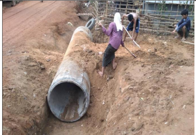
Drainage siphon installation
