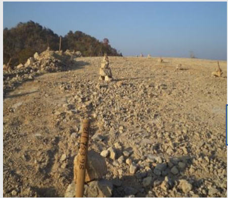
2. Setting out drill pattern
