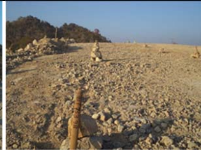
2. Setting out drill pattern
