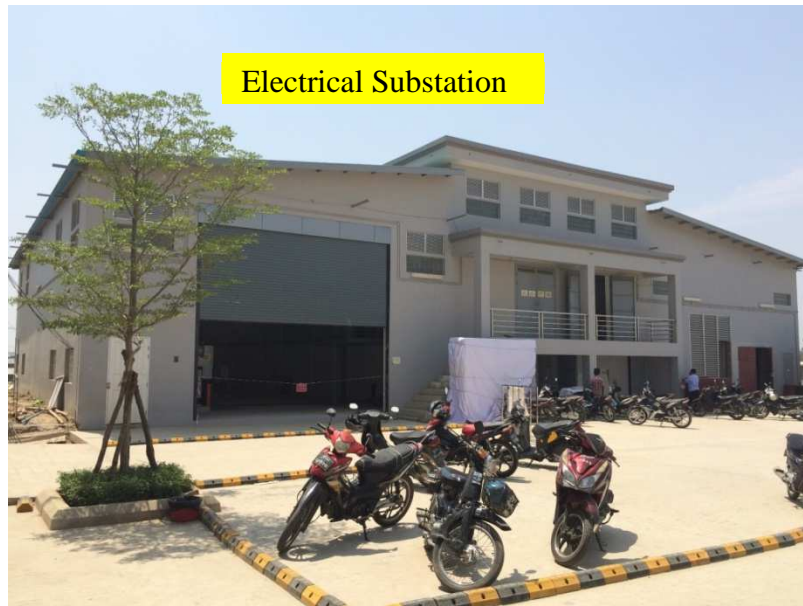
Figure 2.4 Electrical Substation for Mingalar Mandalay Complex
