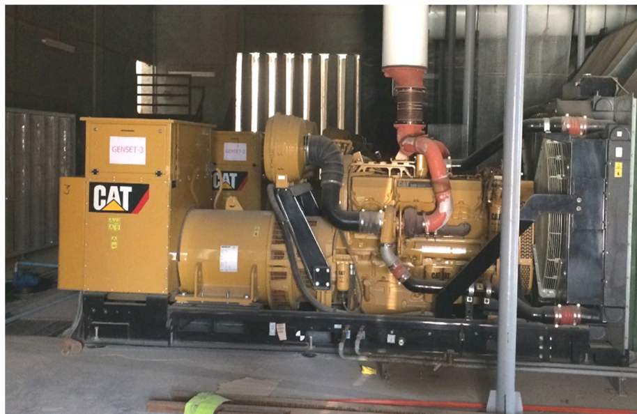
Figure 2.5 Standby Generator
