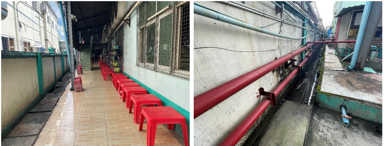
Figure 1-14 Drainage System Photo
