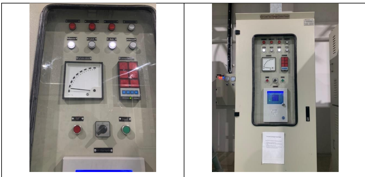
Figure 3-34 Photo of On Load Tap Changer
