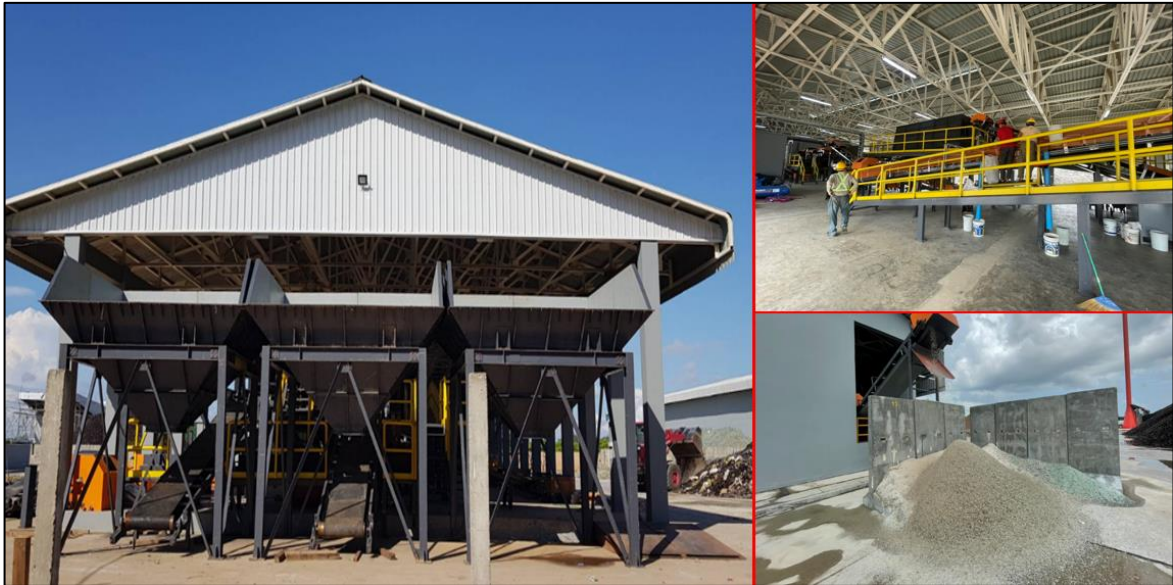
Figure 3-18 Cullet Treatment Plant
