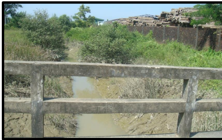
Figure 3. 8 Nearest Creek from the Project Site
