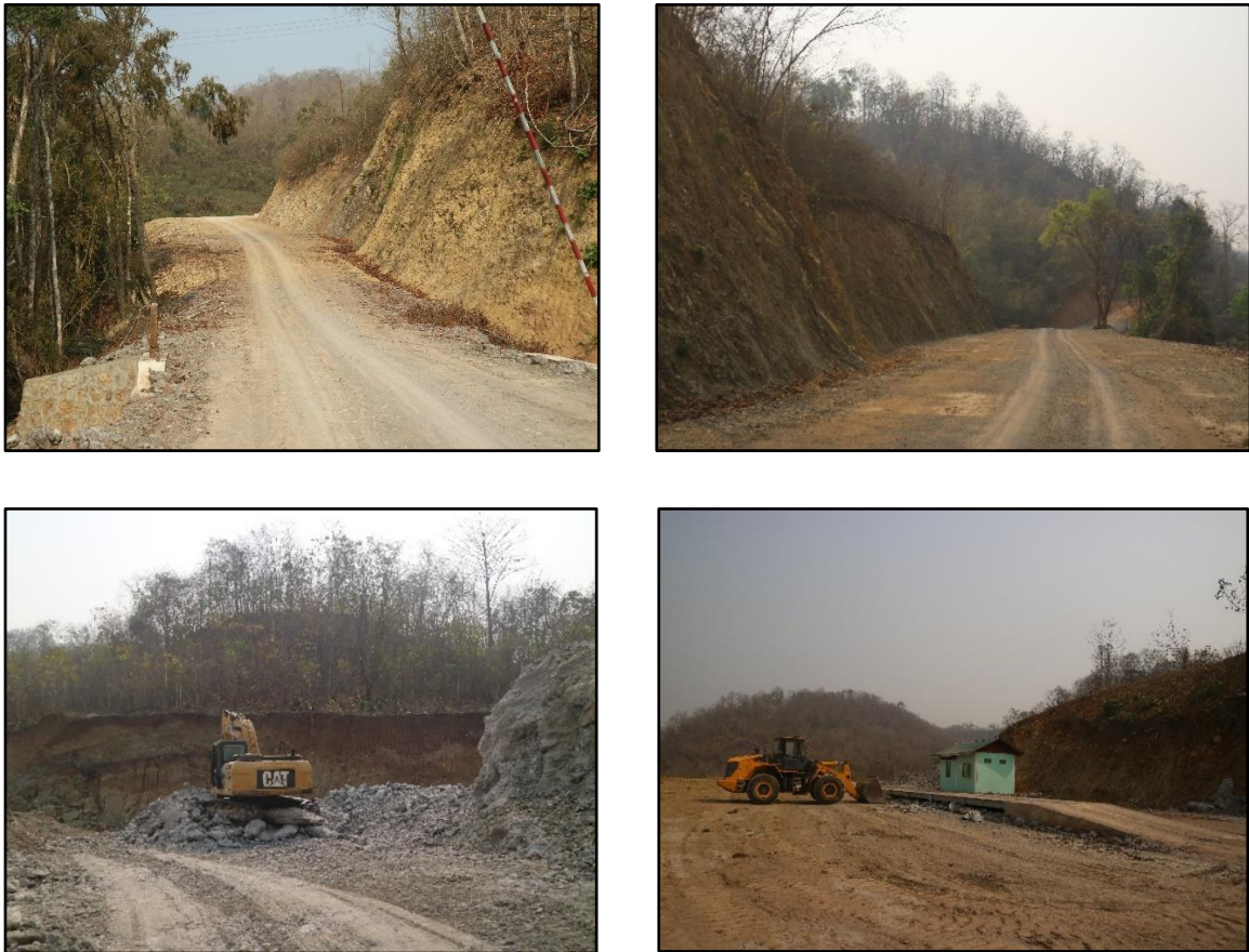
Figure 4.3 Construction Activity of Gypsum Mine
