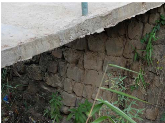
Plate 5.54 Stone abutments of the old Chinese bridge beneath the modern concrete bridge
