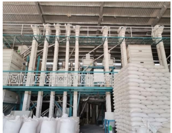
Product Storage Area
