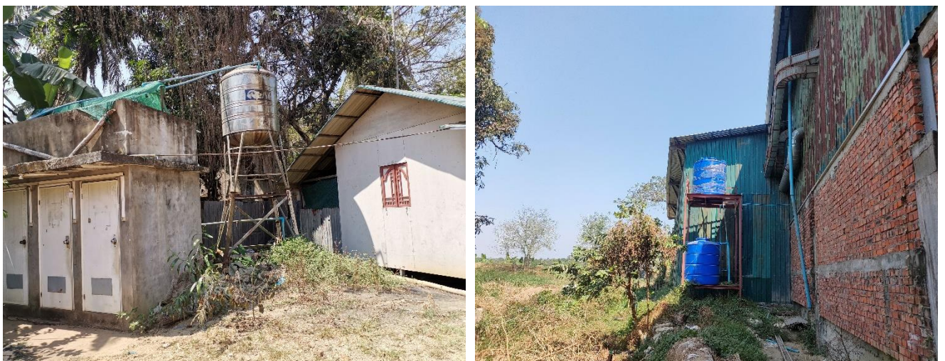
Figure 1-10 Water Storage of Proposed Project
