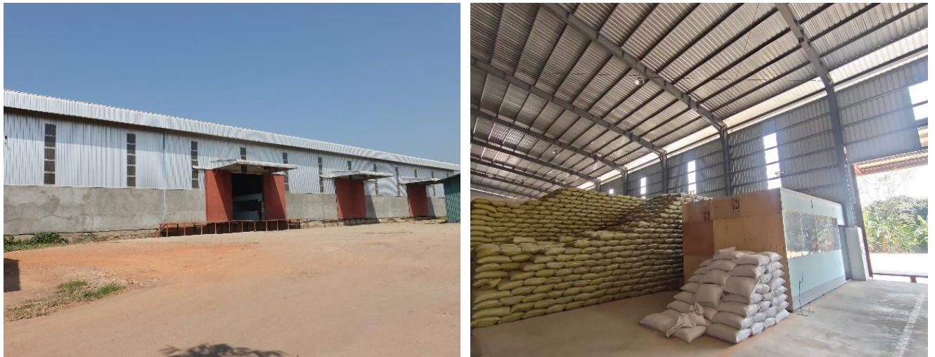
Figure 1-14 Ventilation system implementation photo
