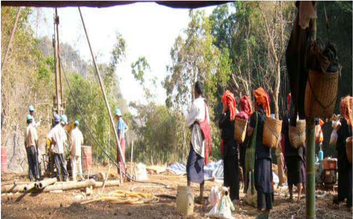
Photo(1) Drilling operation at BH3 drill site.
