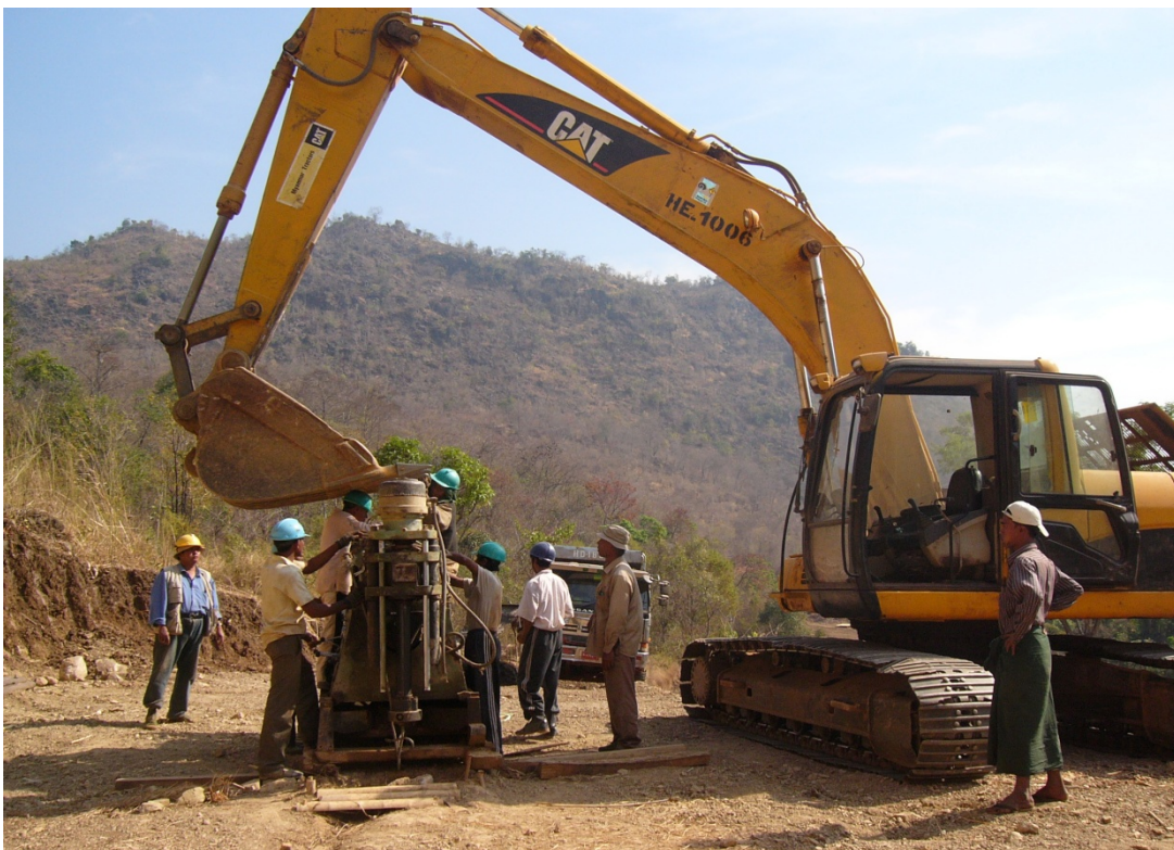
Photo(2) Drill site mobilization from BH2 to BH3 drill site.
