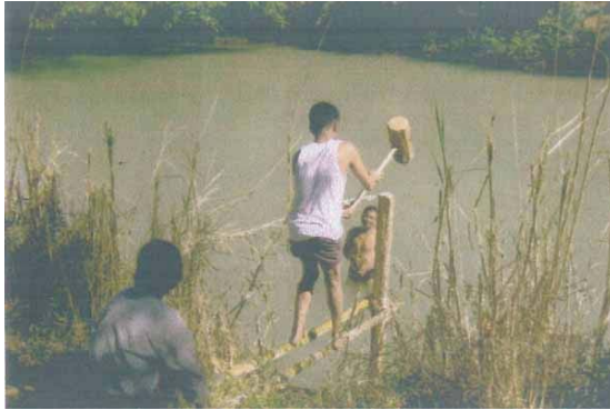
Installation of Staff Gauge at Indein by MGC
