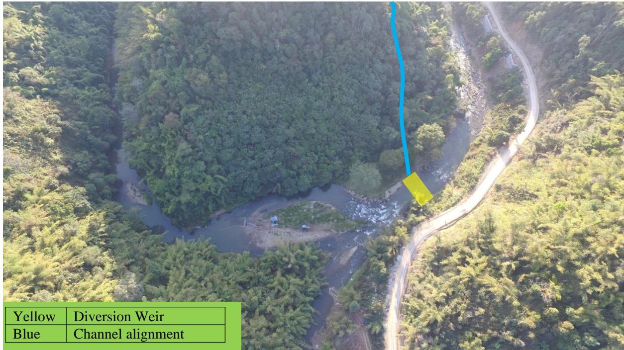
Proposed Diversion Weir Location
