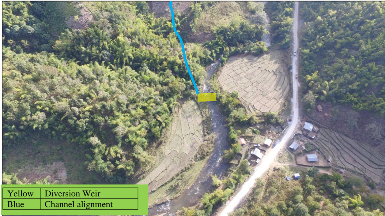
Proposed Diversion Weir Location
