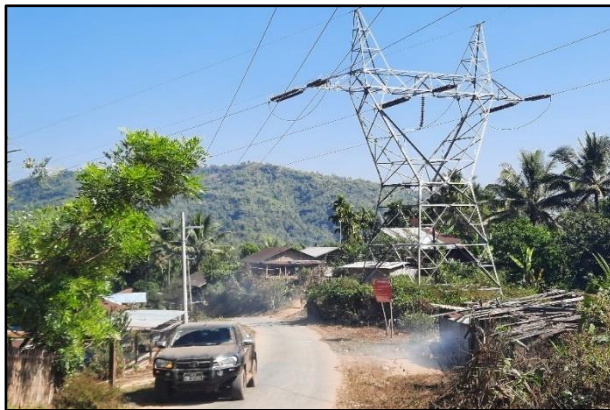
Existing Transmission Tower in Ma Sa Village
