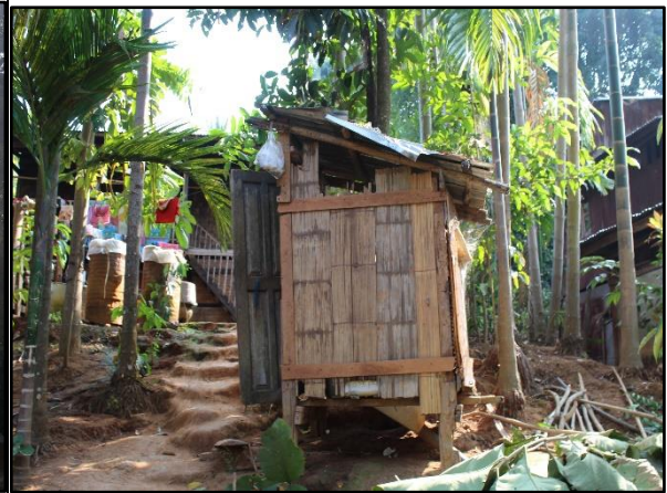
Pit Latrines at Village
