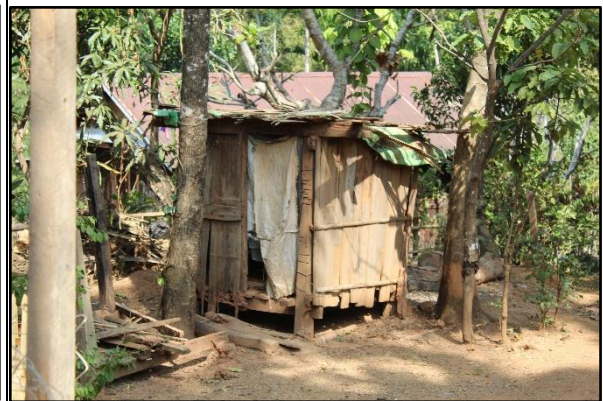
Pit Latrines at Village
