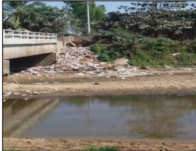
Plate 5.16: Rubbish in the Small Unnamed Creek near the Sabakywe Substation
