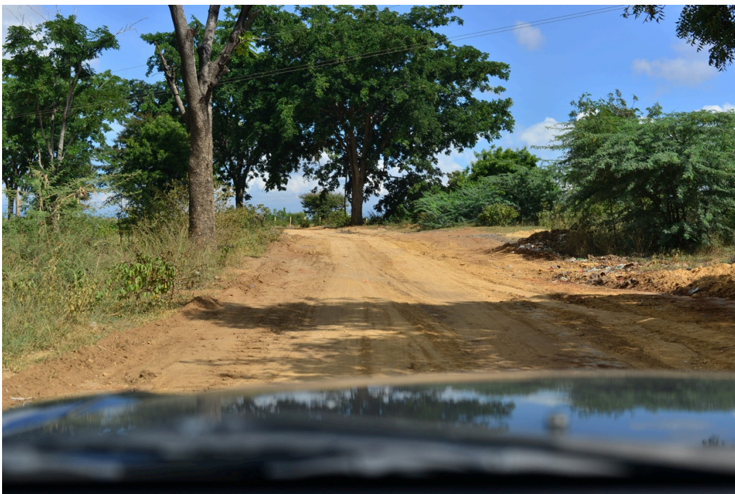
Site entrance located directly off Meiktila-Wundwin Highway
