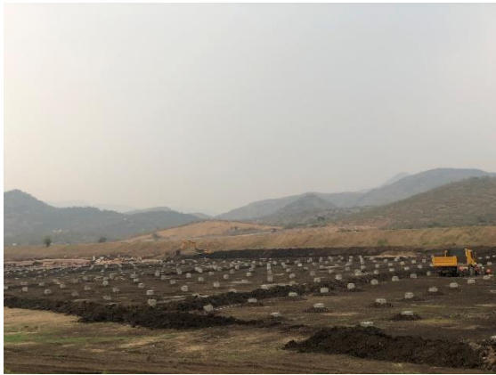
Tracking Bracket Foundations Construction
