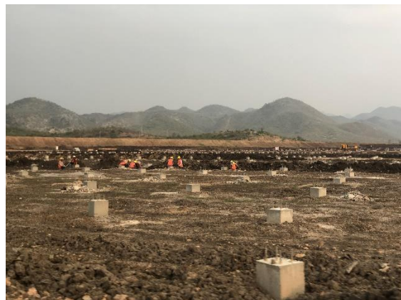
Tracking Bracket Foundations Construction
