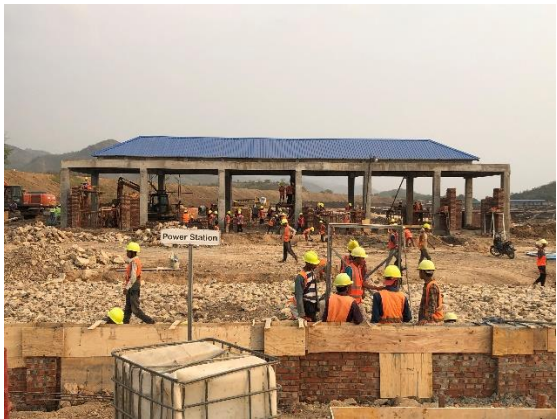
Power Station Construction
