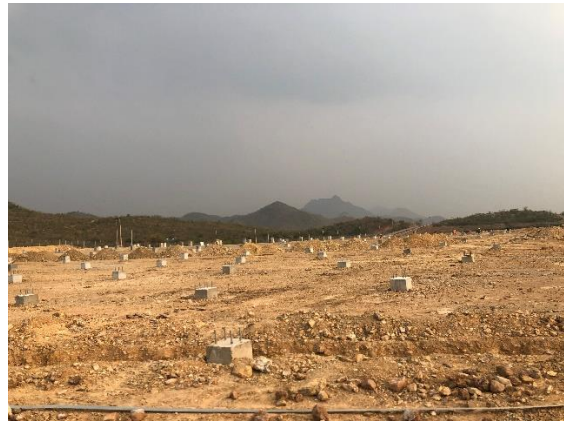
Tracking Bracket Foundations Construction
