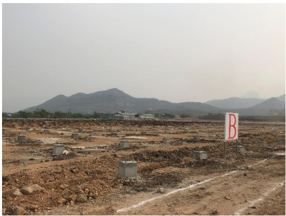
Tracking Bracket Foundations Construction
