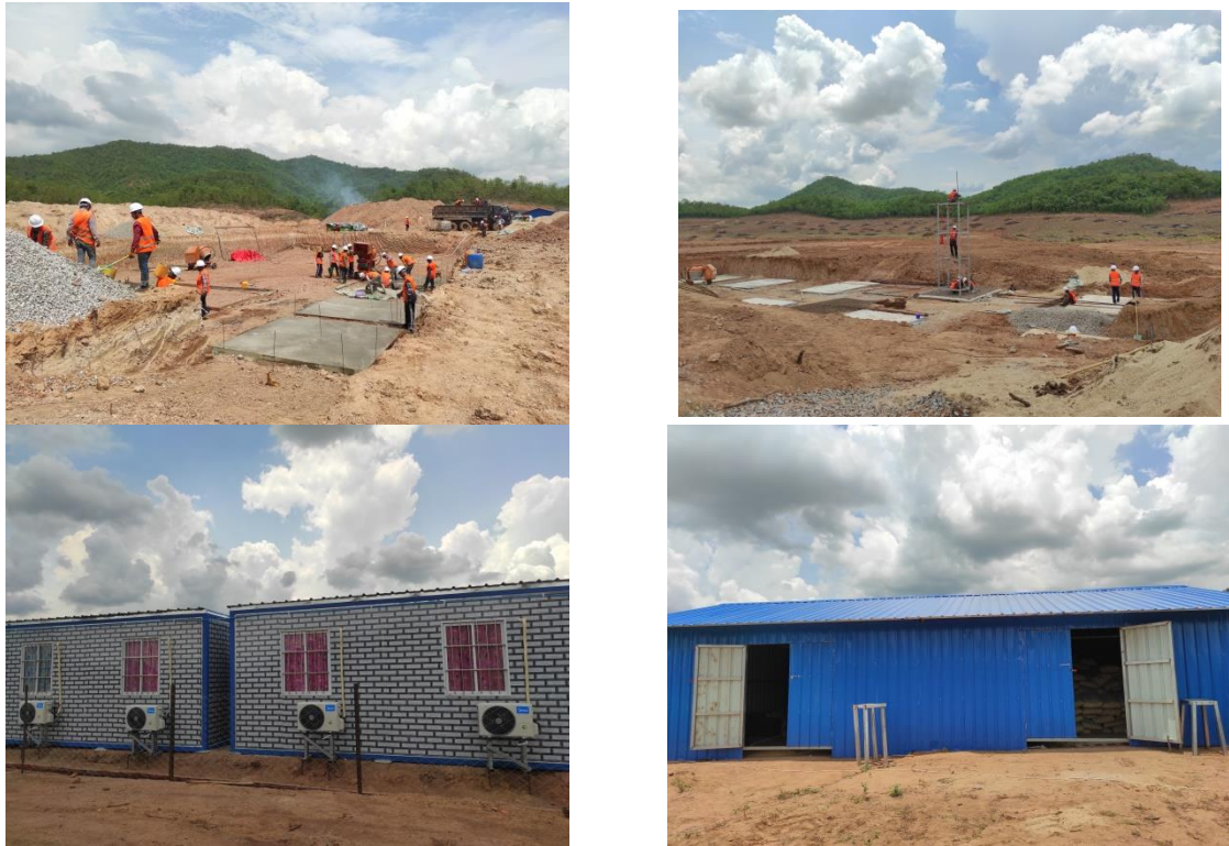
Figure 2.18 Current Site Condition
