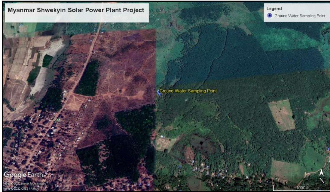
Figure 6.13 - Location of Ground Water Quality Sample Taking Point
