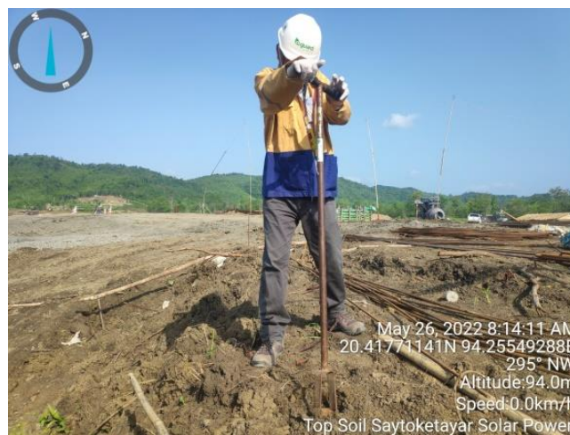
Figure 6. 14 Getting Soil Sampling within site area
