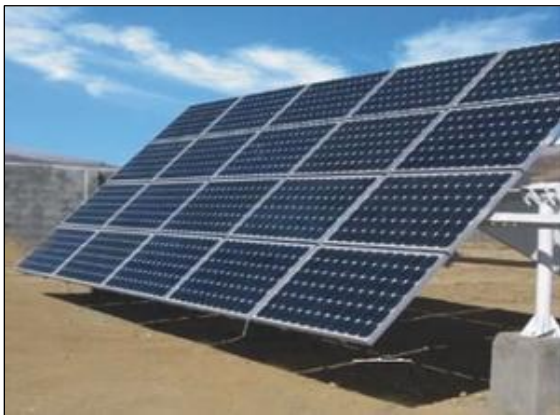
Figure 2.8 Horizontal Single-Axis Bracket Type
