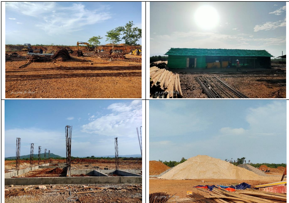
Figure 2.17 Current Conditions of Project Site
