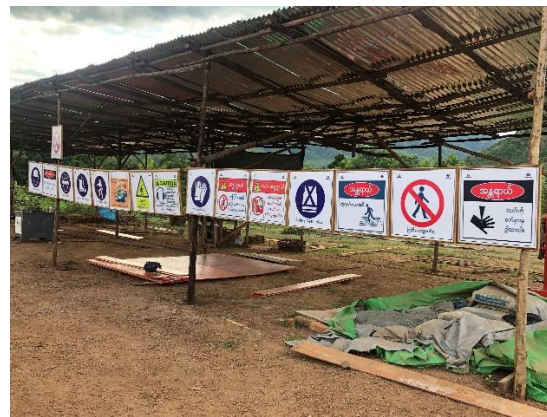
Construction Activities Working Area
