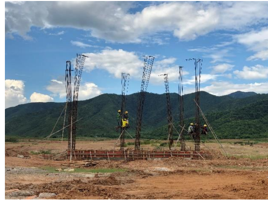
Guard House Construction
