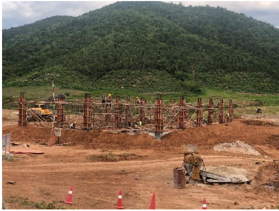
Control Building Construction at Switchyard
