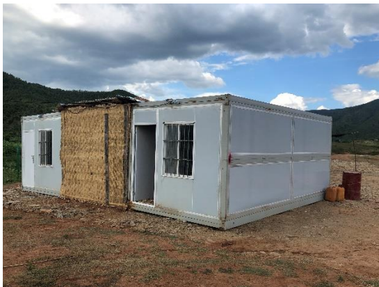
Temporary Project Office
