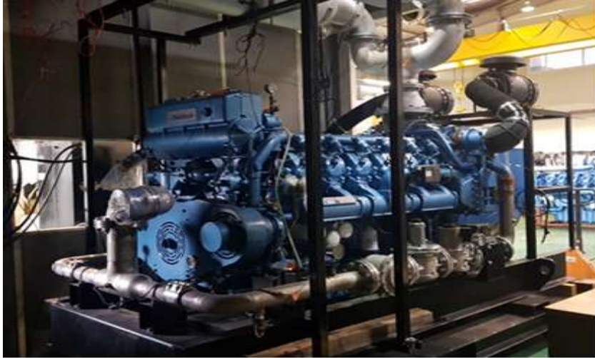
500 kW LFG Generator (Operating time : 1day X 3 hr ~ 5 hr)
