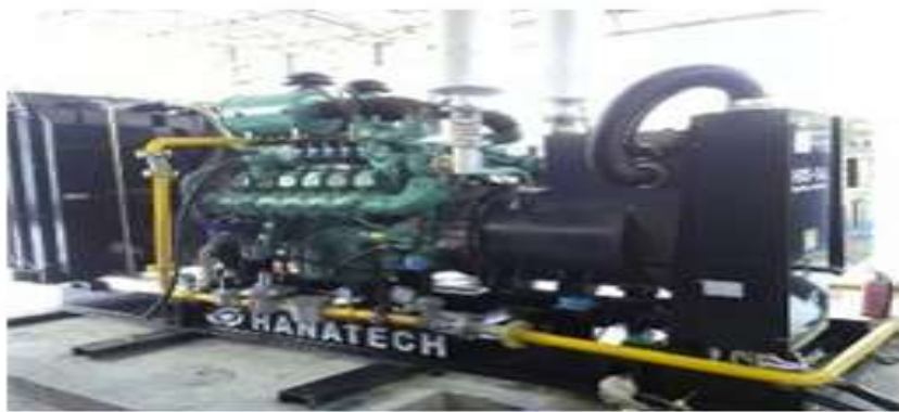
500 kW LFG Generator (Operating time : 1day X 3 hr ~ 5 hr)
