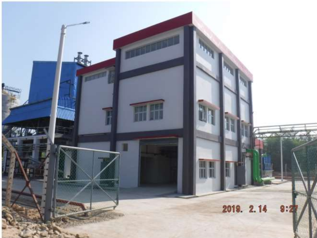
(a) Power House Building
