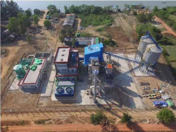
Project Completion Overall View
