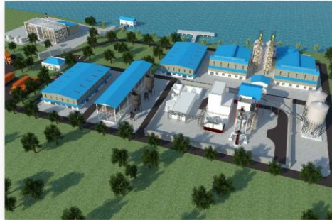
1.8 MW Gross Rice Husk Fired BTG Power Plant Project Myaung Mya
