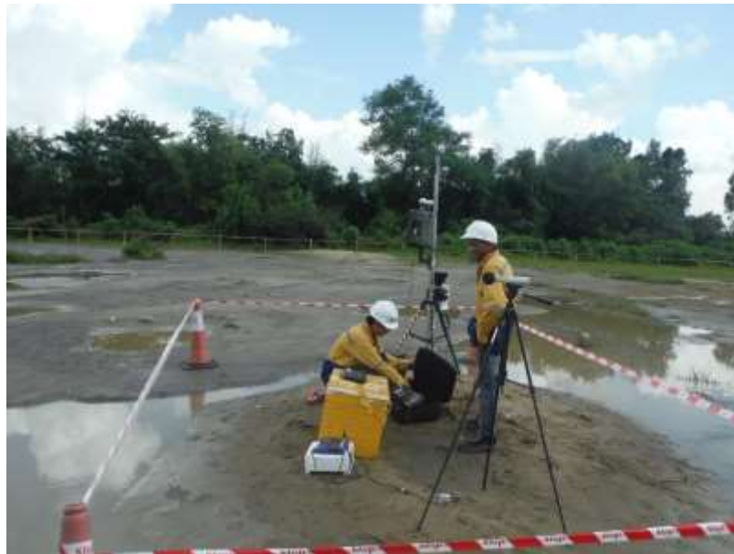
Figure 4. 9 Vibration level Measurement at the project site
