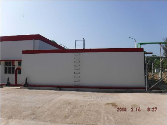
Project Completion Photo Raw Water Reservoir
