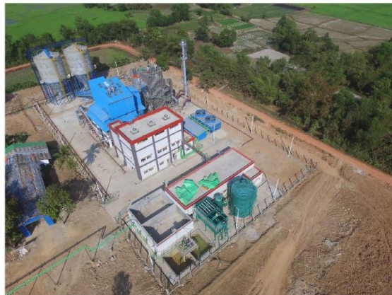
Project Completion Overall View
