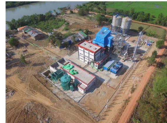
Project Completion Overall View
