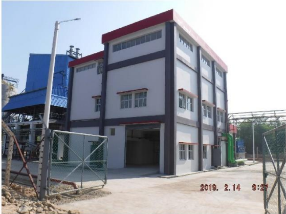
Project Completion Photo Power House Building
