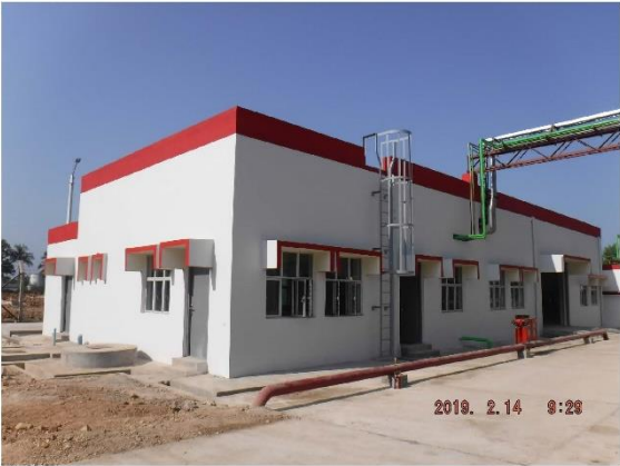
Project Completion Photo Water Treatment Plant Building
