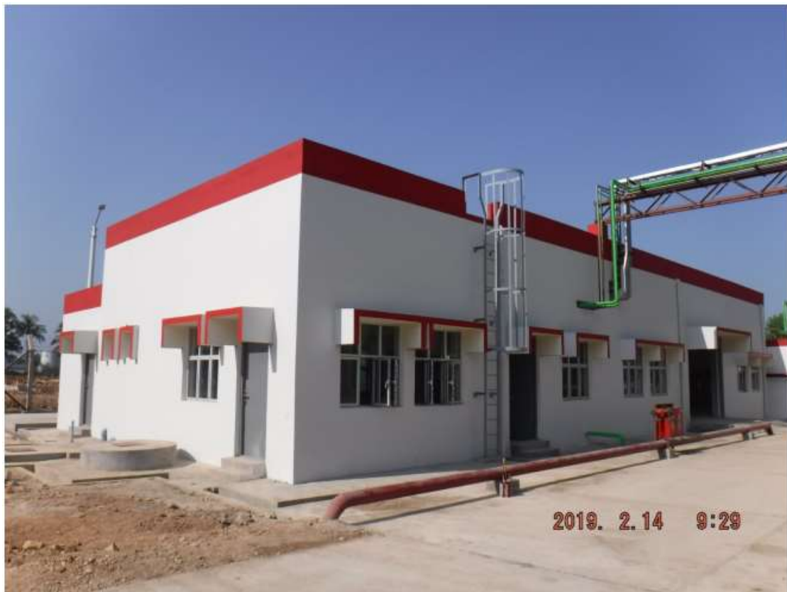
(b) Water Treatment Plant Building
