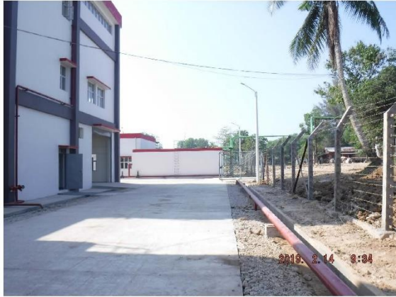
Project Completion Photo Road Completion
