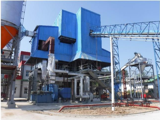
Project Completion Photo Boiler House Building
