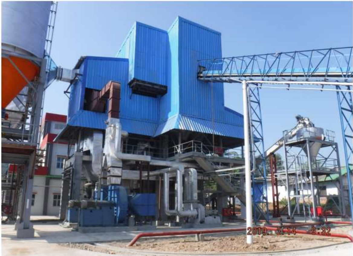
(c) Boiler House Building
