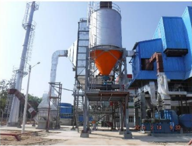
Project Completion Photo Fly Ash Silo
