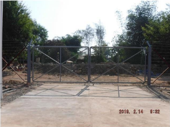
Project Completion Photo Fence & Gate
