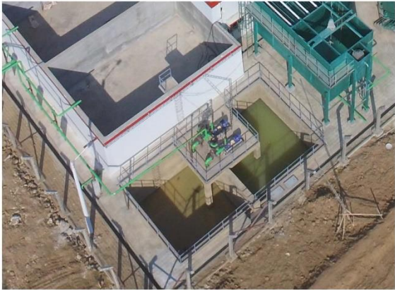
Project Completion Photo Guard Pond
