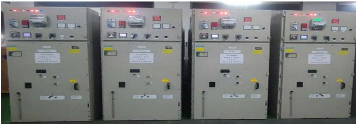
33kV Vacuum-circuit breaker
