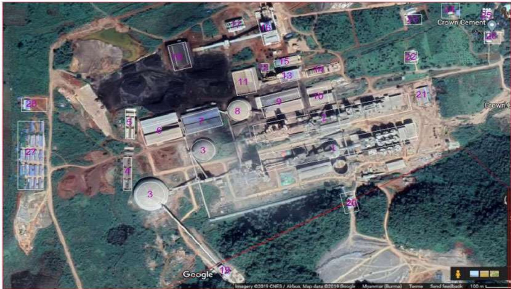
Figure – 4: Overview of Crown Cement Factories (4000 ton factory and 1000 ton factory) and coal-thermal plant (The 60W- Boiler Turbine (thermal plant) which is the theme of this EIA report)
