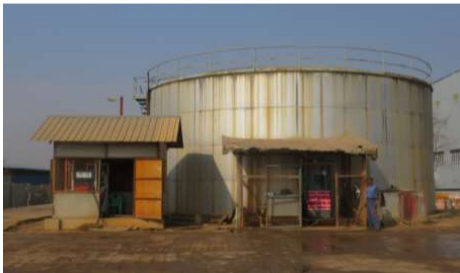
Figure – 44: Fuel oil depot
