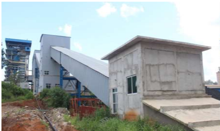
Figure – 13: Coal conveyor
