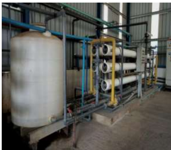
Figure – 51: R.O Membrane System
