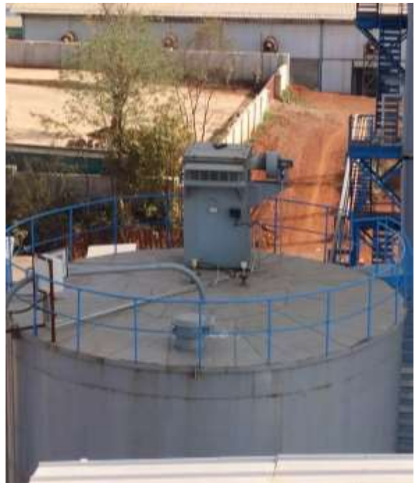
Figure – 23: Bag Filter and Limestone Silo
