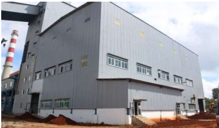
Figure – 12: Turbine house
