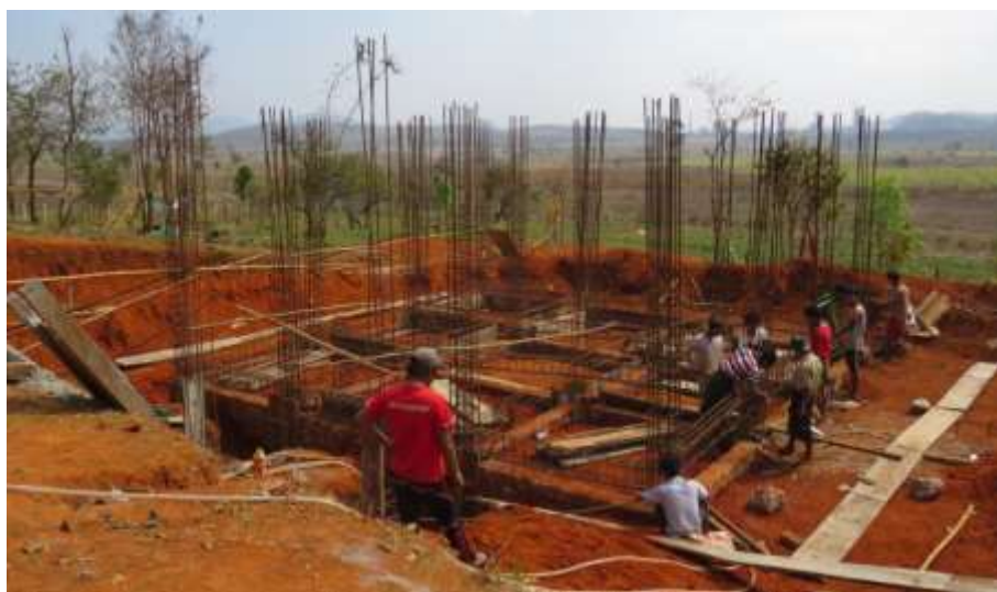
Figure – 108: Construction of Khe San Village pagoda
