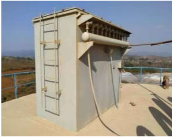
Figure – 24: Bag Filter (Fly Ash Silo)
