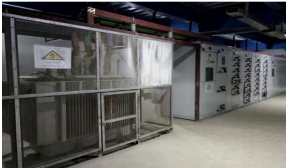
Figure – 38: High voltage control panel
