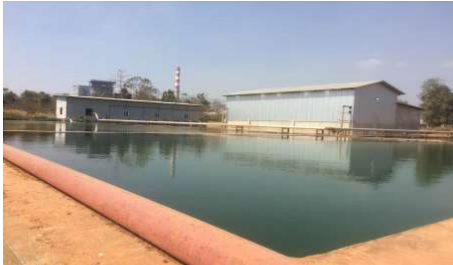
Figure – 49: 1.5 million gallons water tank
