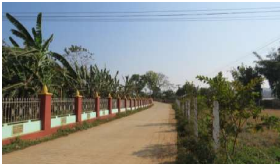
Figure – 93: The village concrete road constructed by the company
