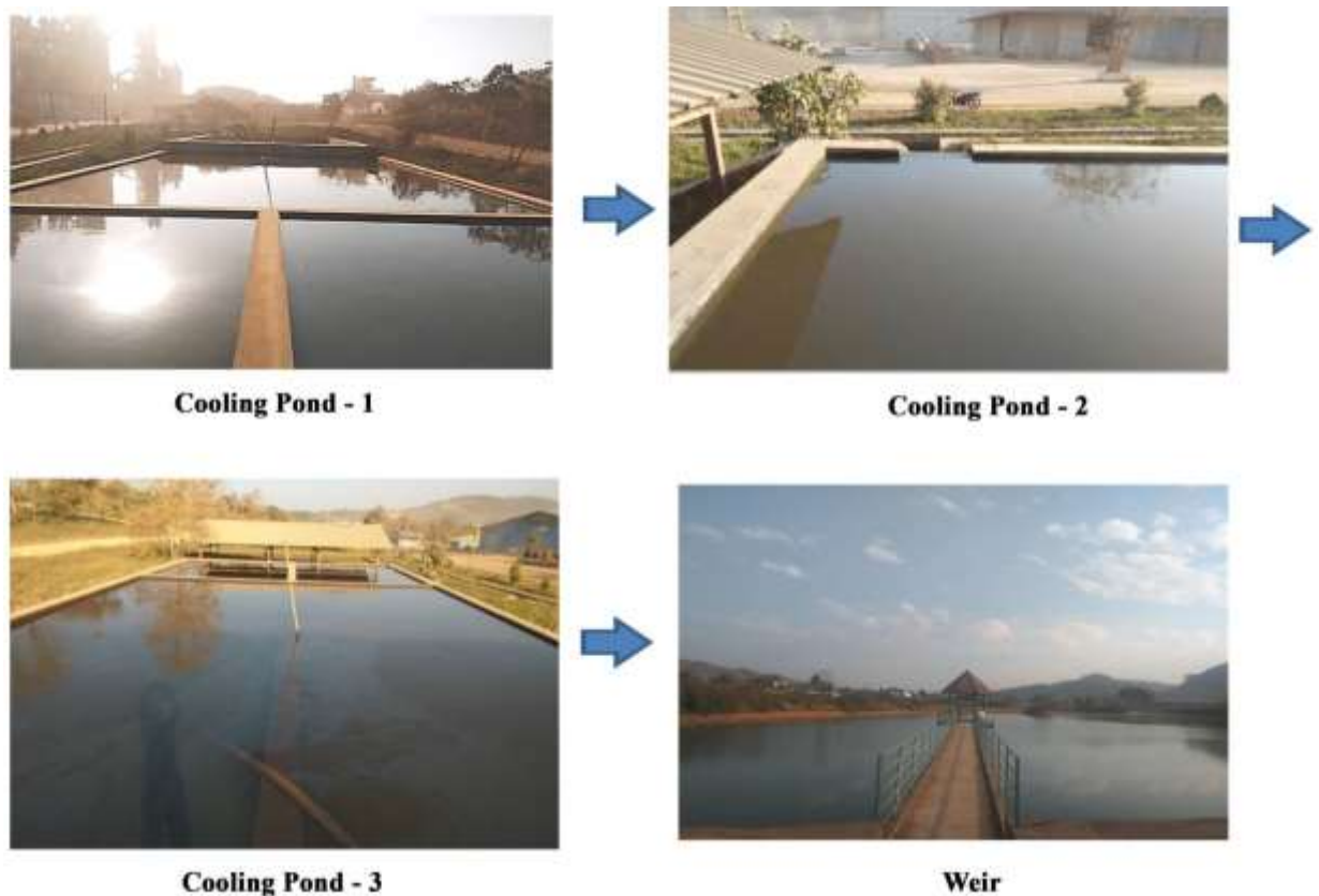
Figure – 70: Recirculation of used water system from 4 cooling tanks
