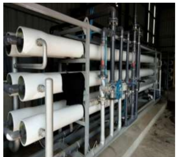
Figure – 51: R.O Membrane System
