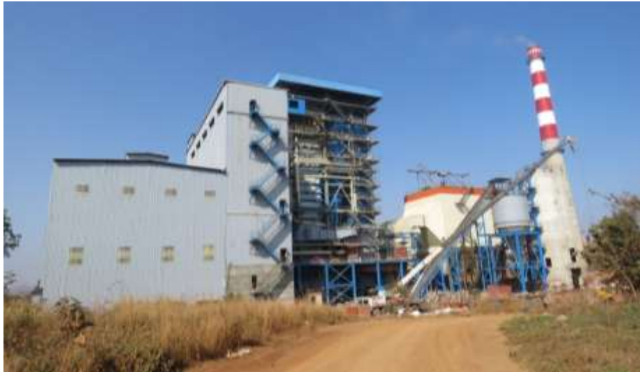
Figure – 9: Coal thermal plant in the process of construction
