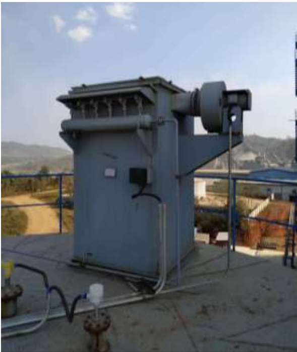
Figure – 23: Bag Filter and Limestone Silo
