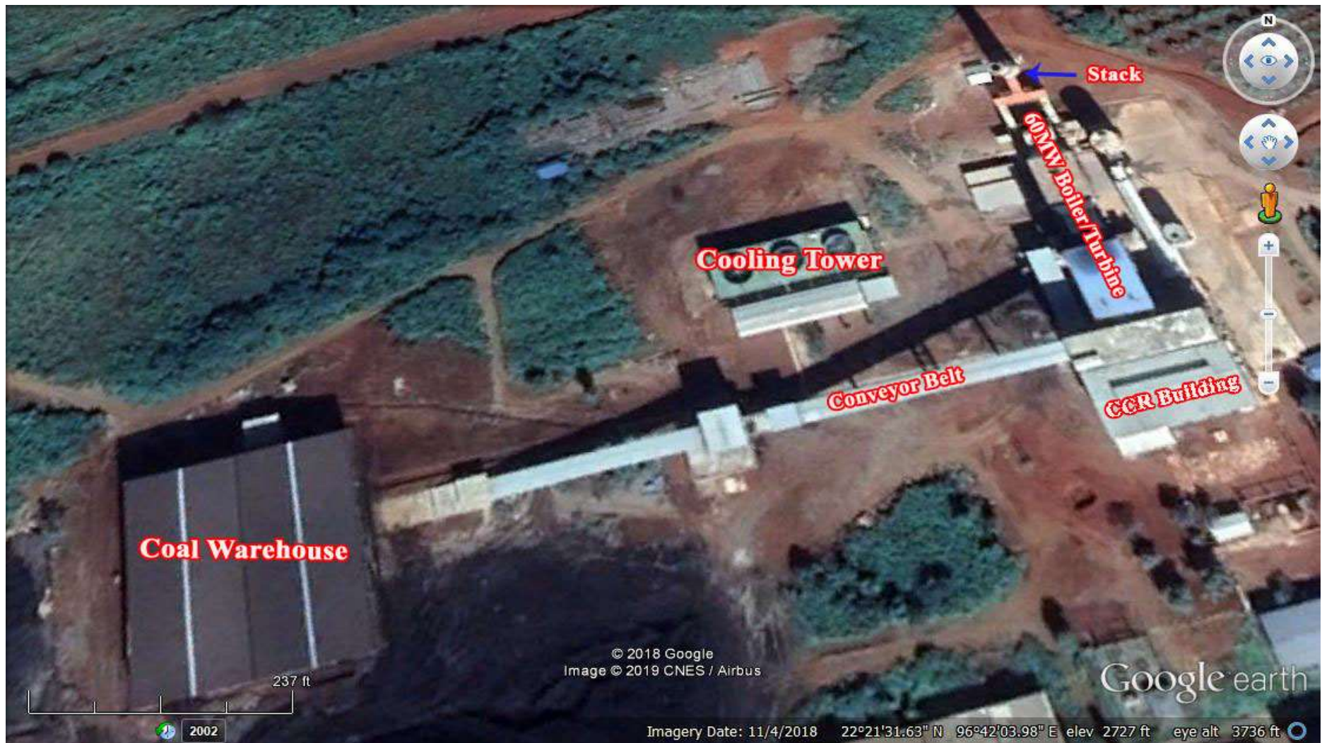
Figure – 5: Satellite image of the proposed project site (in the north-eastern portion of the main cement factory compound)
