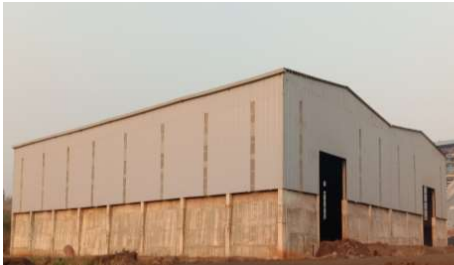
Figure – 17: Coal storage
