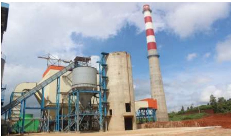
Figure – 30: Bottom ash silo and stack
