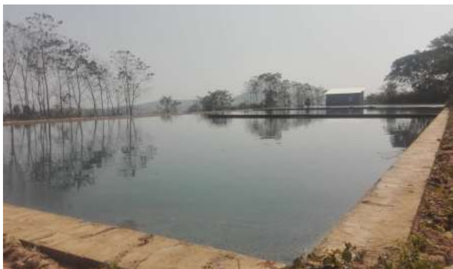
Figure – 48: 2.1 million gallons water tank
