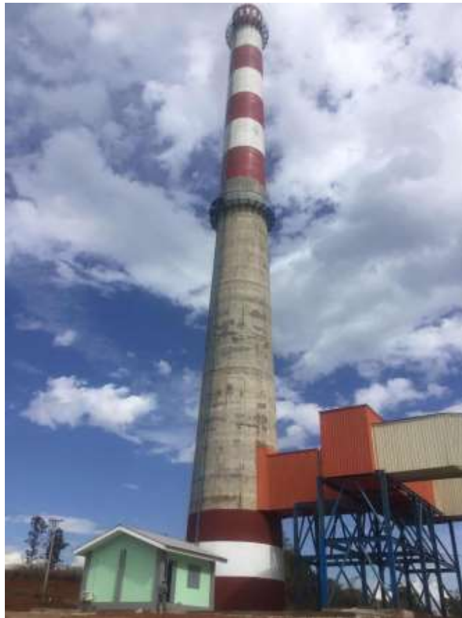
Figure – 31: Stack (83.8 m) and gas analyser house
