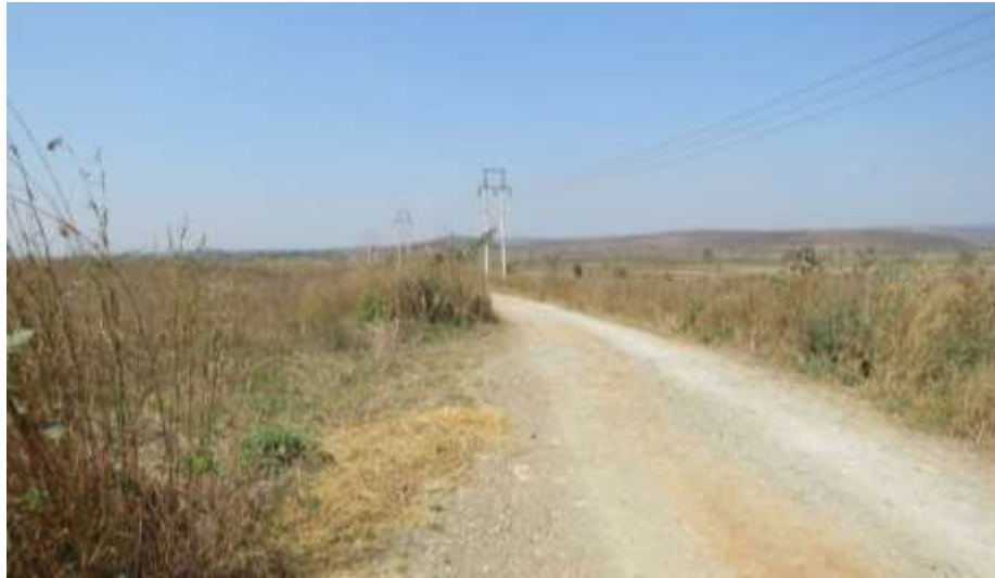
Figure – 100: The village road constructed by the company
