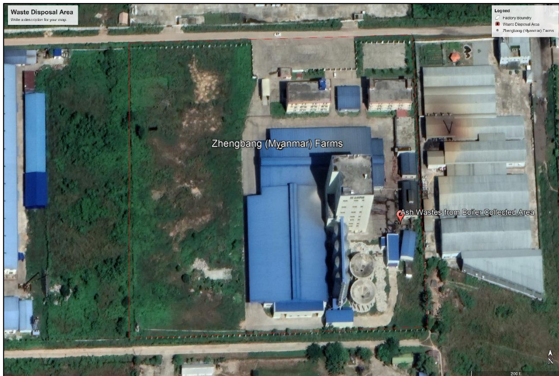
Figure 6-4: Temporary Ash Wastes Storage Area
