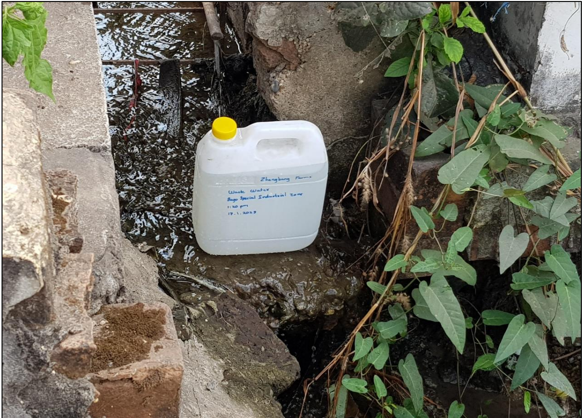
Figure 6-5: Drainage Outlet of the Factory
