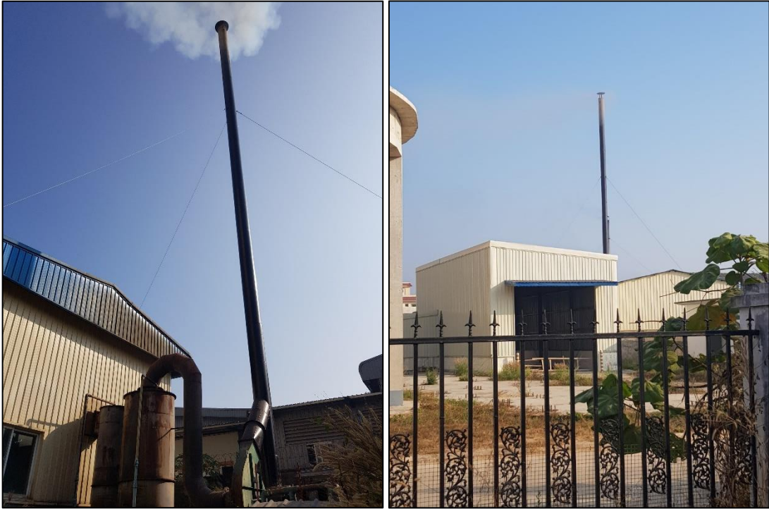
Figure 6-2: Stack of the Boiler
