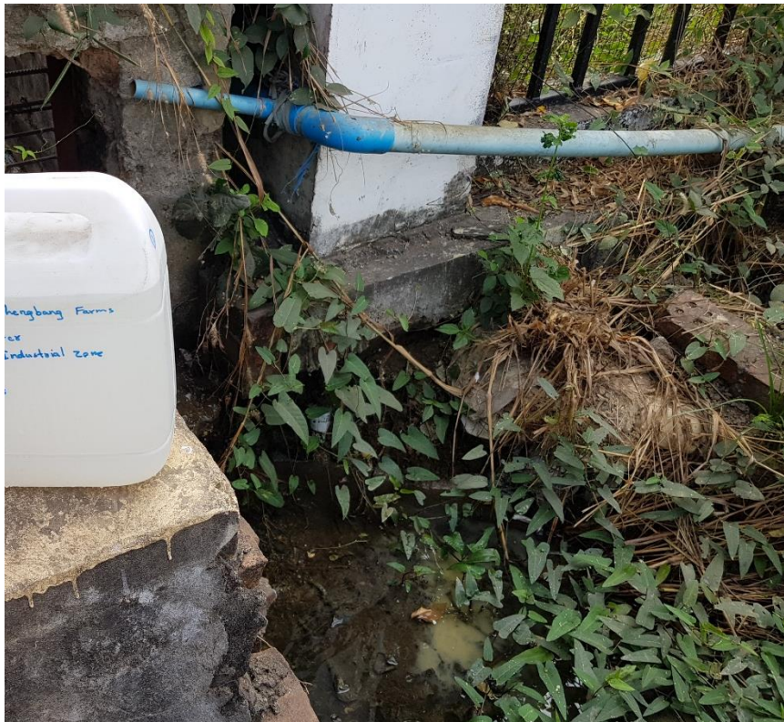
Figure 4-11: Edge of Drainage (before municipal sewer)
