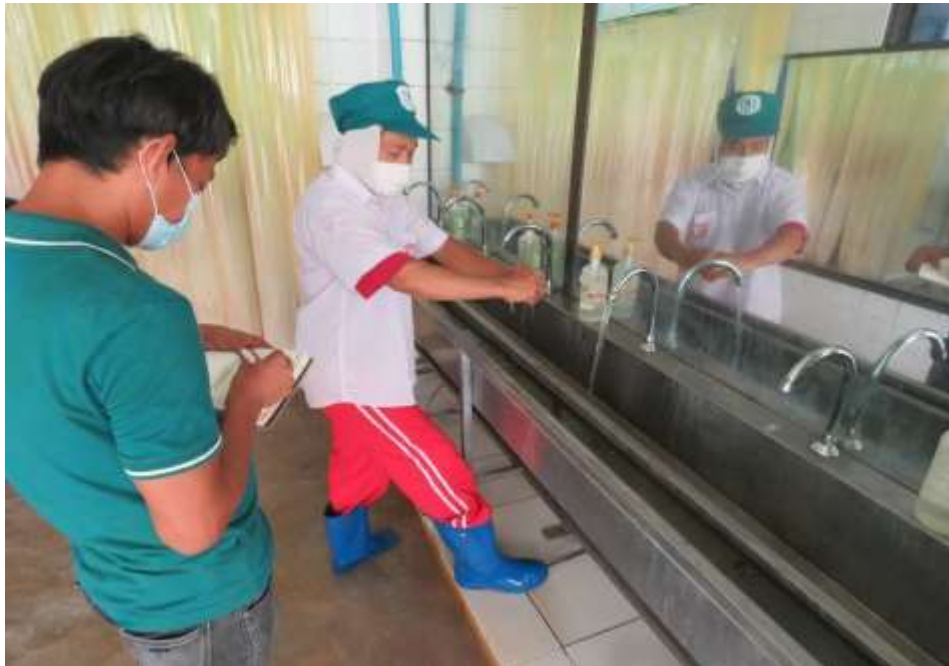
Figure 4. 23 : Sufficient hand and foot washing facilities (Chlorine level for hand washing is 10ppm and foot dip is 100ppm) at the entrance of the processing area
