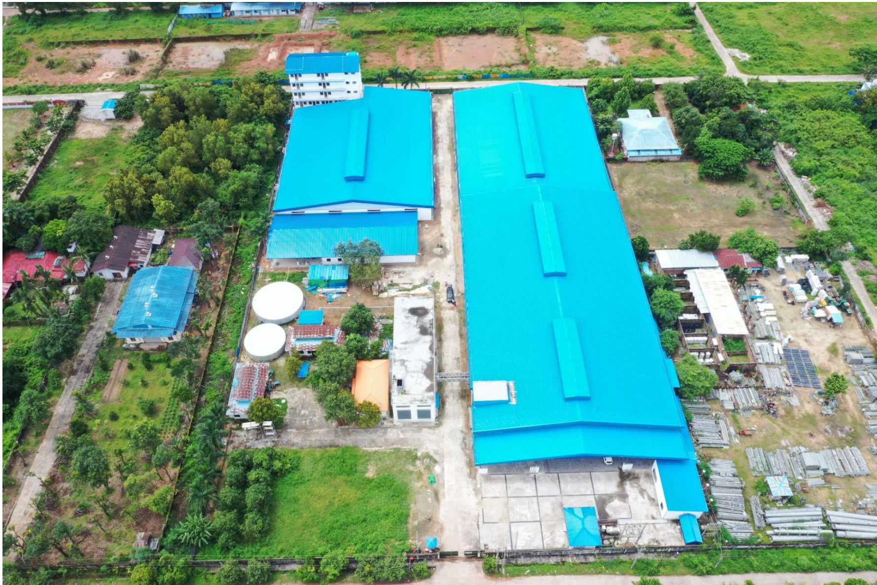
Figure 3-10 Aerial of Photo of Project (September 2022)
