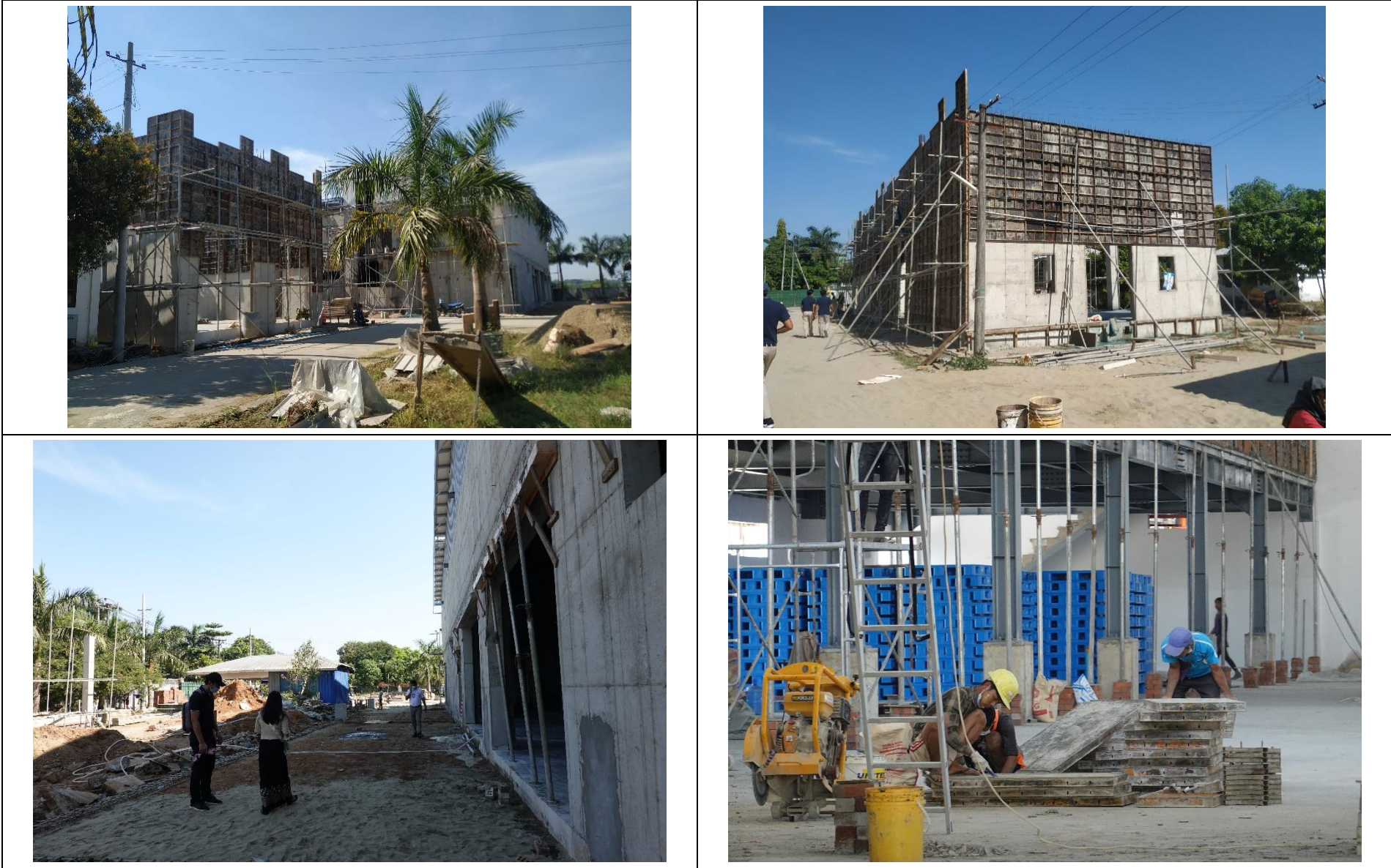
Figure 3-11 Project Site Photo in December 15, 2020
