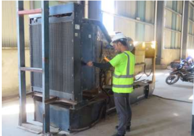
Figure – 83: Measuring vibration at project site
