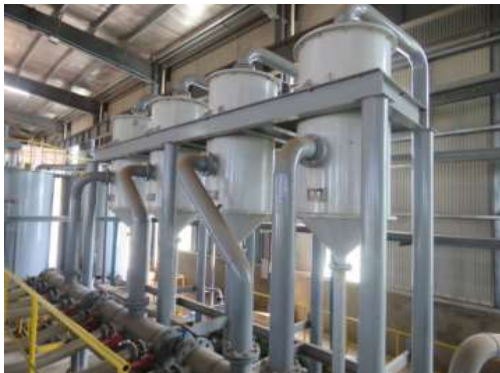
Figure-40: Water, air separators
