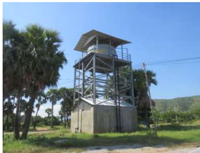
Figure-55: Ground concrete tank and overhead tank for industrial use
