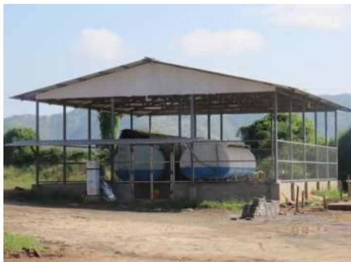
Figure-59: Fuel depot
