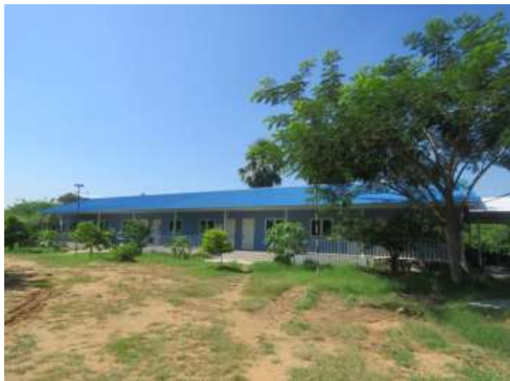
Figure-17: Housing for technicians
