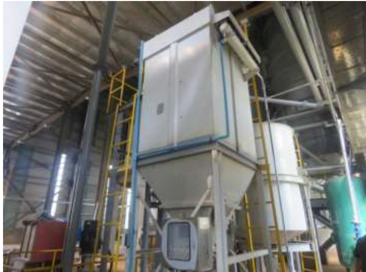
Figure-35: Bag filter unit
