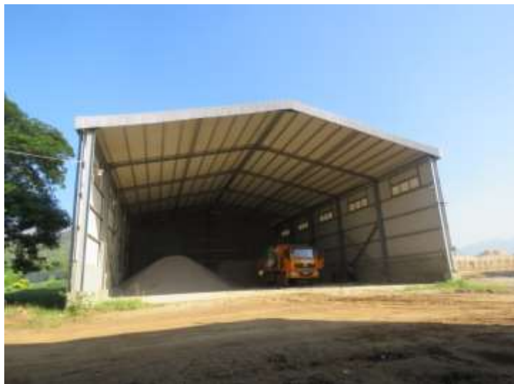
Figure-15: Warehouse for raw material
