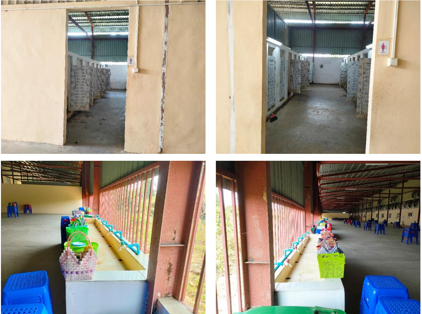
Figure 3-14 Toilet Facilities Photos
