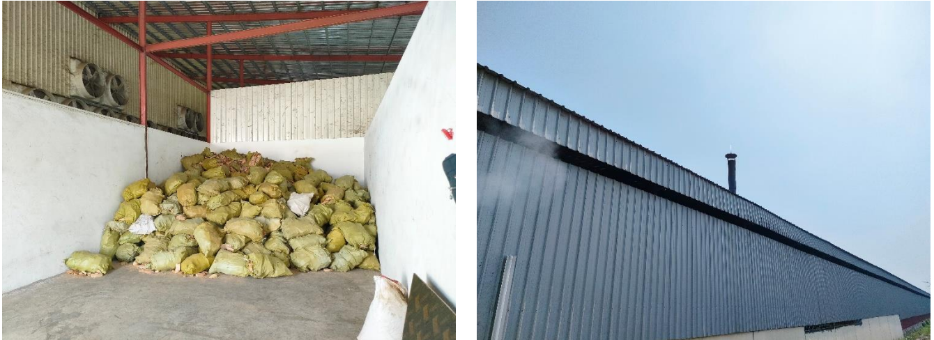
Figure 3-9 Installed photo of boiler
