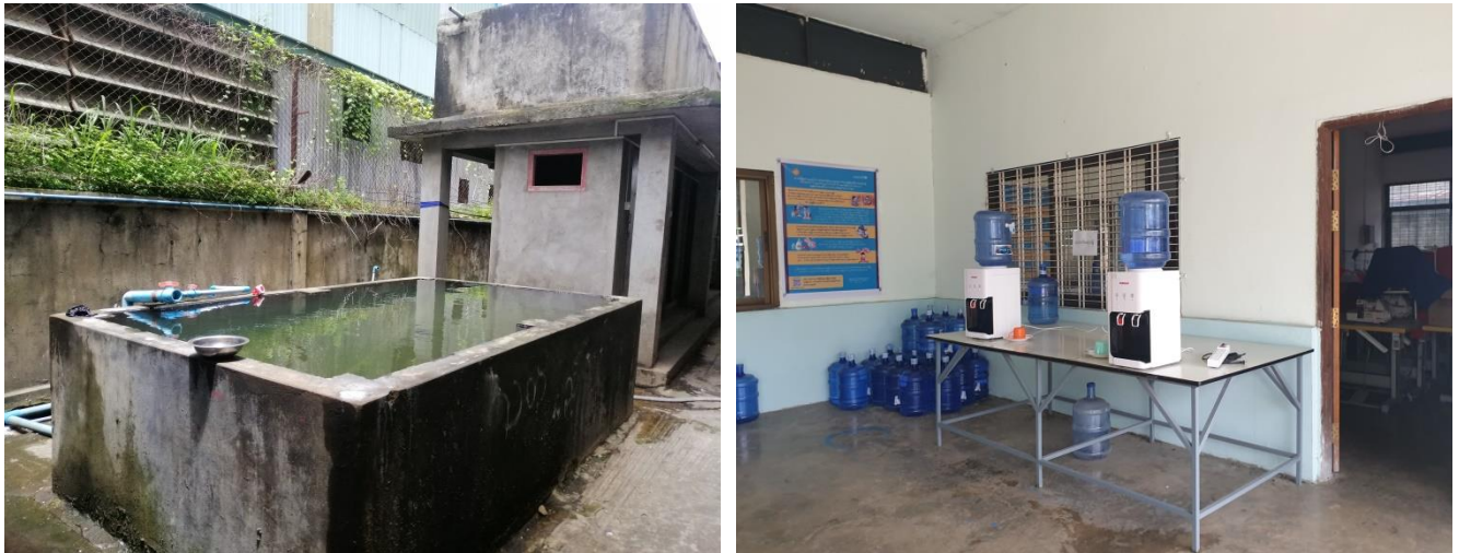
Figure 3-9 Water Supply System Photo
