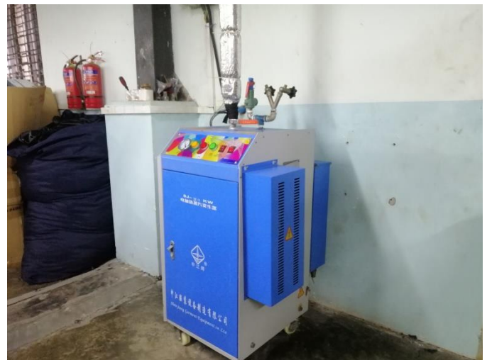
Figure 3-11 Electric Steam Boiler Photo
