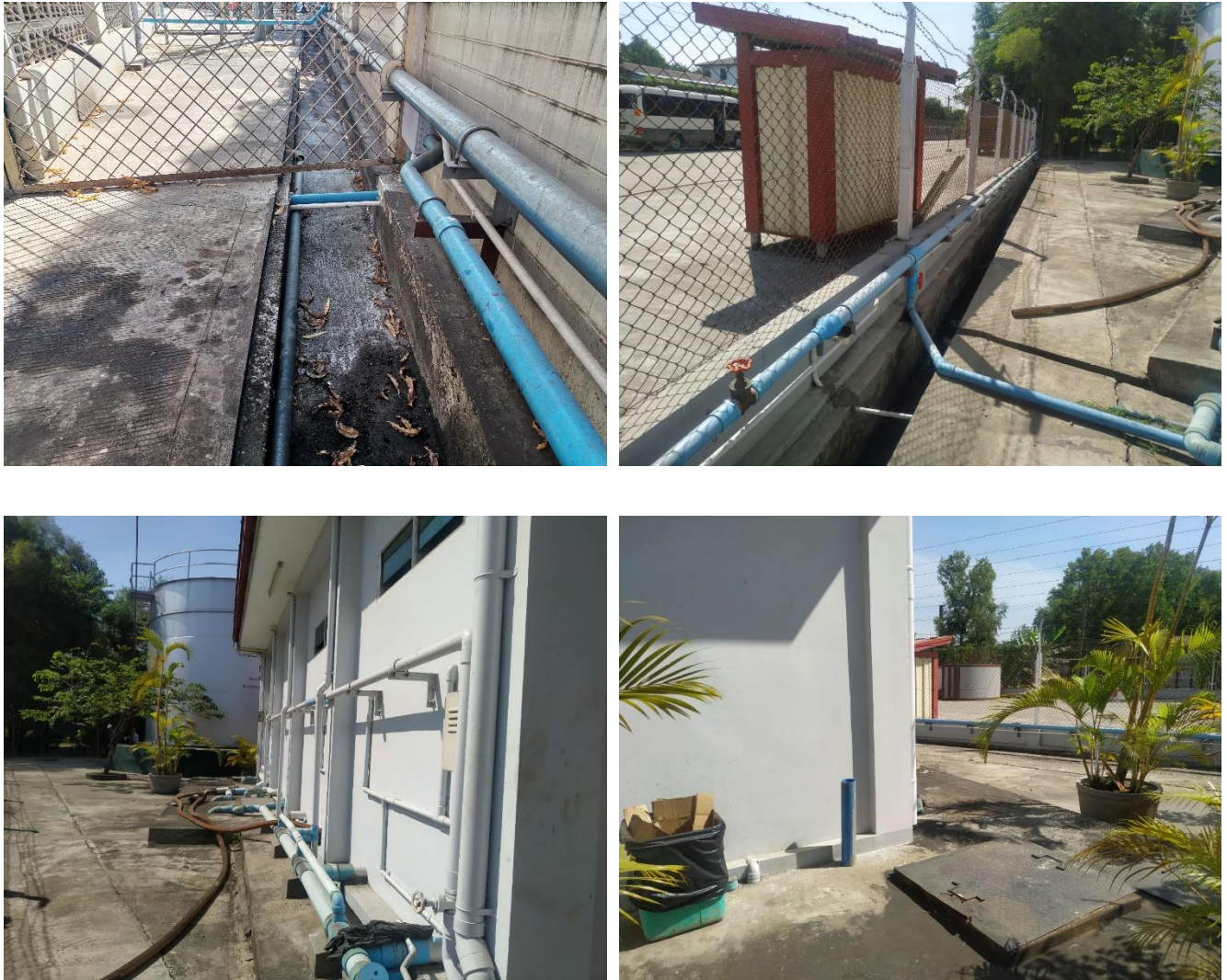
Figure 3-14 Drainage System in Factory Compound
