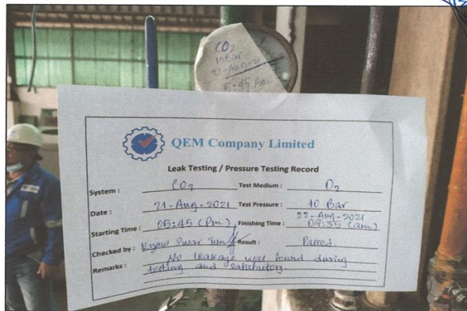
Finishing of Test
