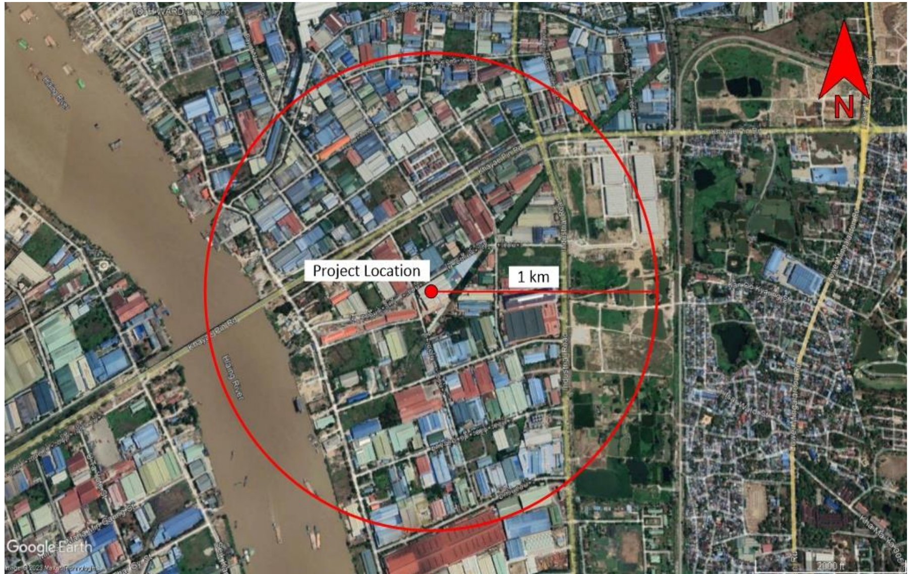
Figure 3-3 Adjacent Map of Min Dhama Steel Structures Company Limited
