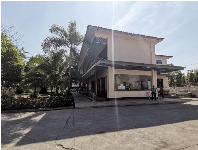
Office & Security Room
