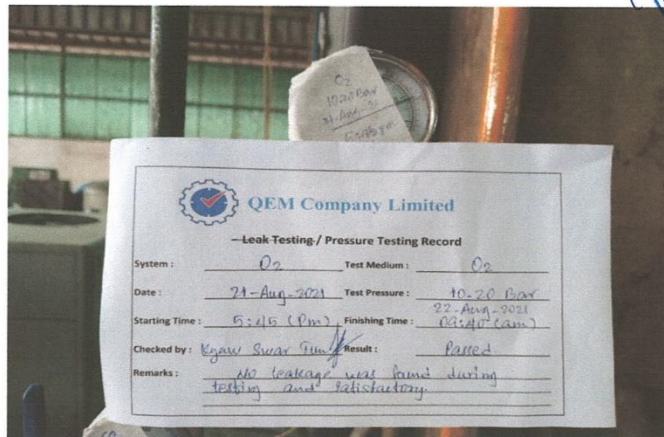
Finishing of Test
