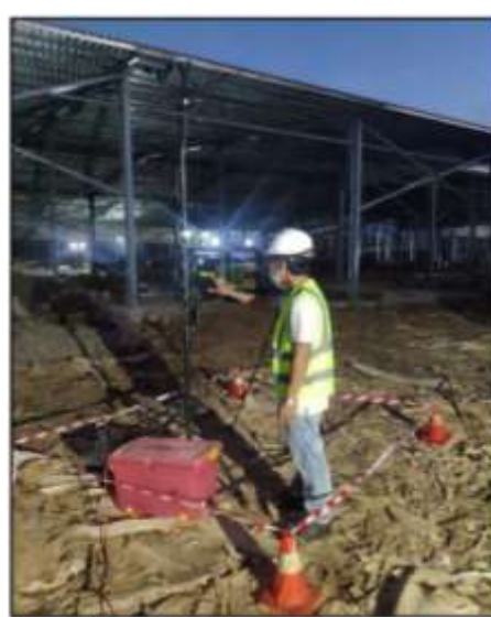
Figure – 22: Measuring air quality at project site during night time
