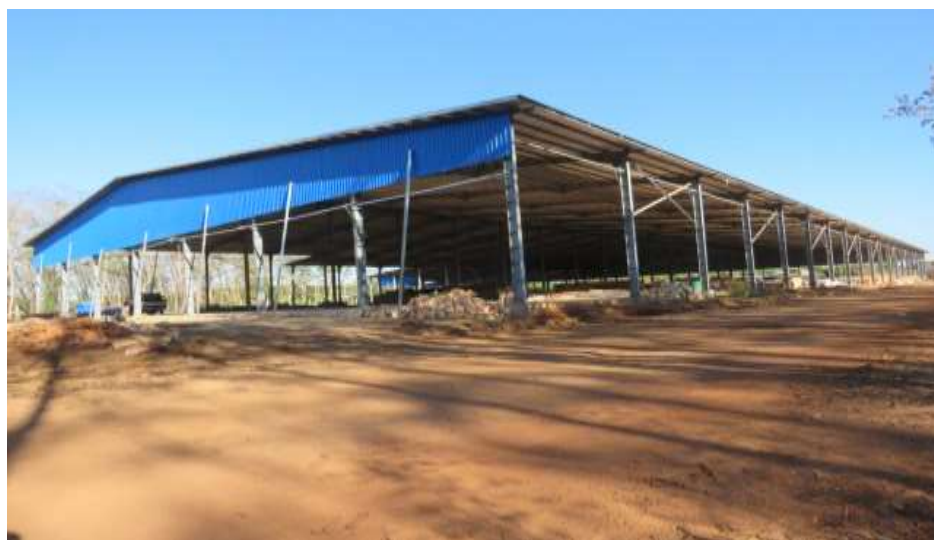
Figure – 11: The factory in the process of construction
