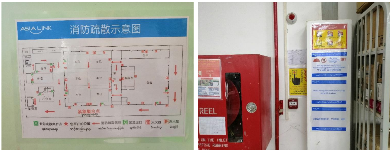
Figure 6-2 Emergency exit layout plan and warning signs
