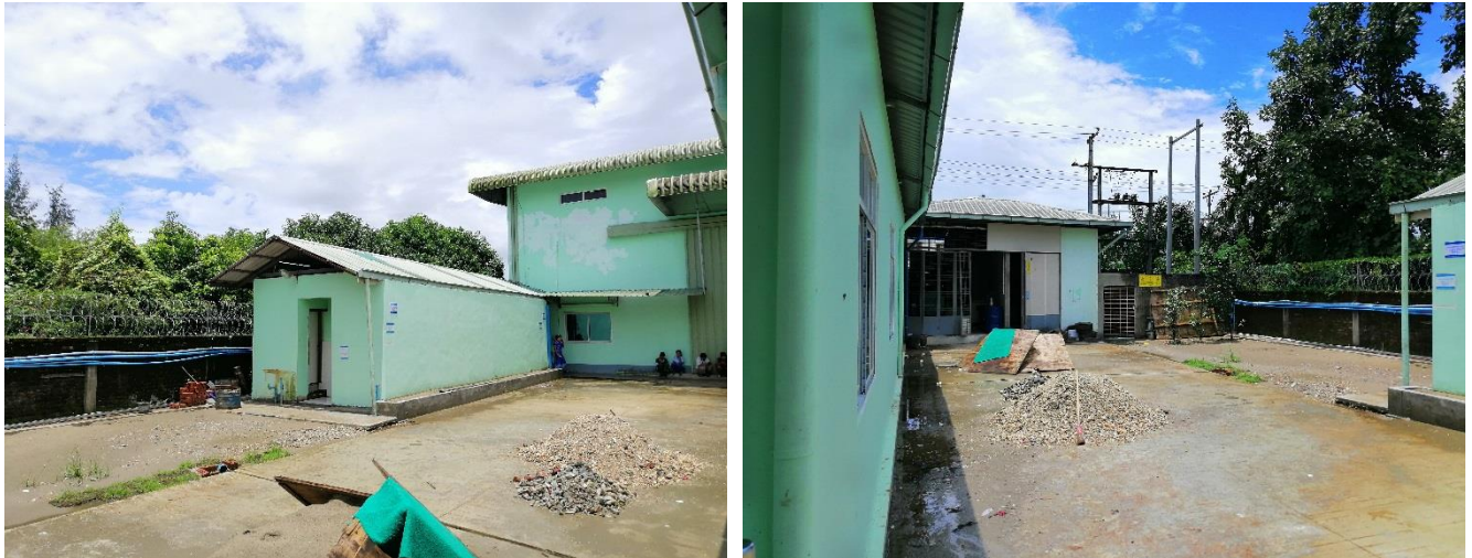
Figure 5-4 Drainage and Septic tank in project area
