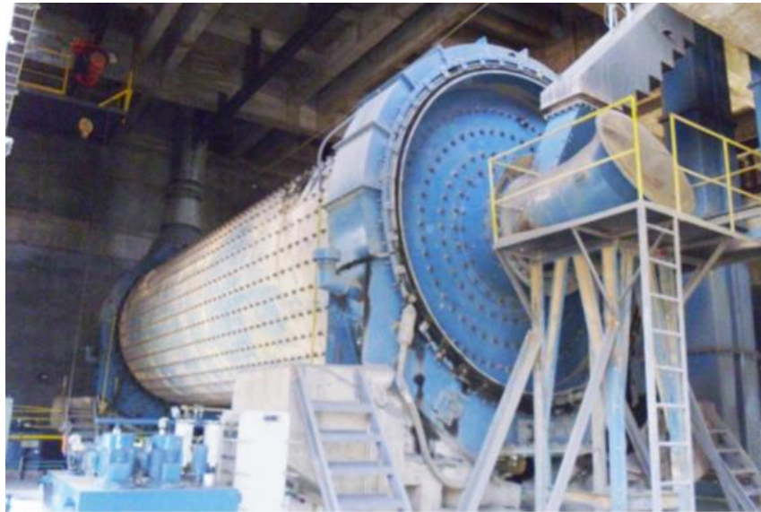
Figure 4.7 Cement Grinding Mill
