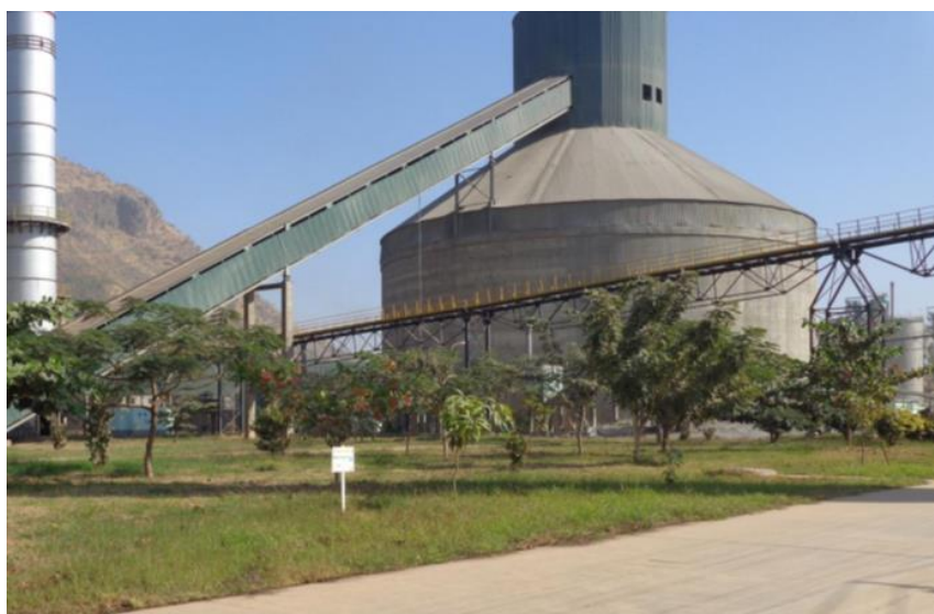
Figure 4.4 Clinker Silo and Conveying System
