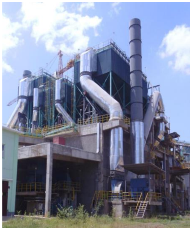
Figure 4.8 Cement Grinding Mill (Press Roller)
