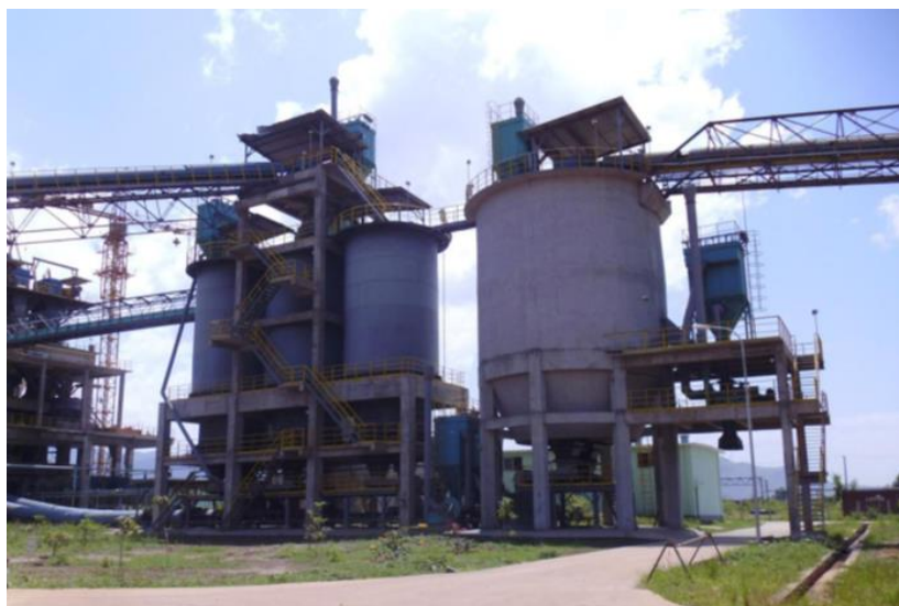
Figure 4.5 Cement Proportioning Station
