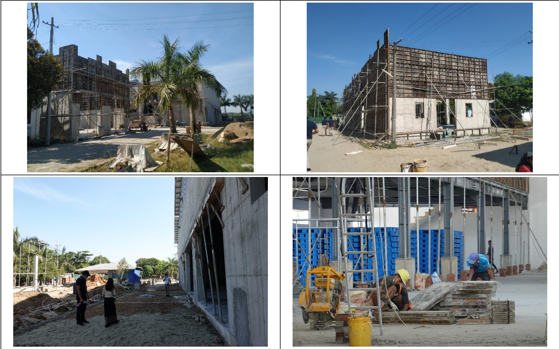
Figure 3-11 Project Site Photo in December 15, 2020
