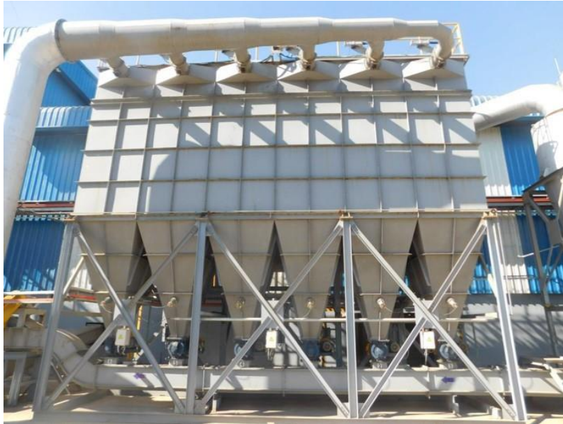
Figure 3.9-4: Filtering Bag House for Lead Dust of Rotary Smelter
