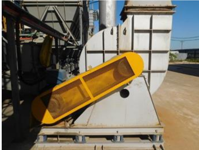
Figure 3.9-6: Dust Line, Blowing Fan and Motor
