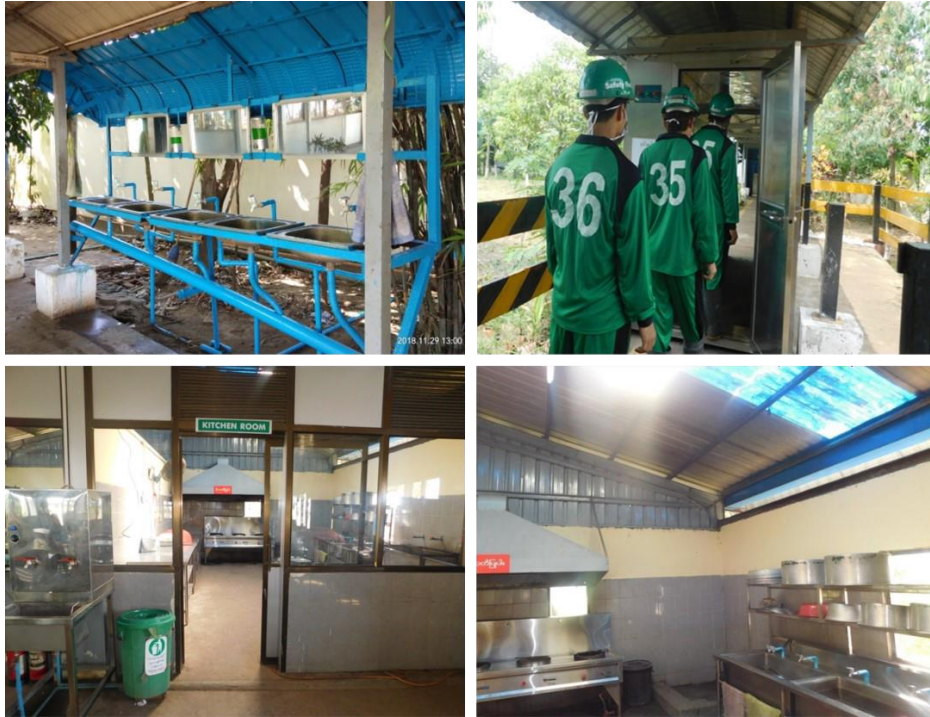
Figure 5.8.10-2: Air Blower Before Kitchen Room, Washing Facilities and Dining Room
