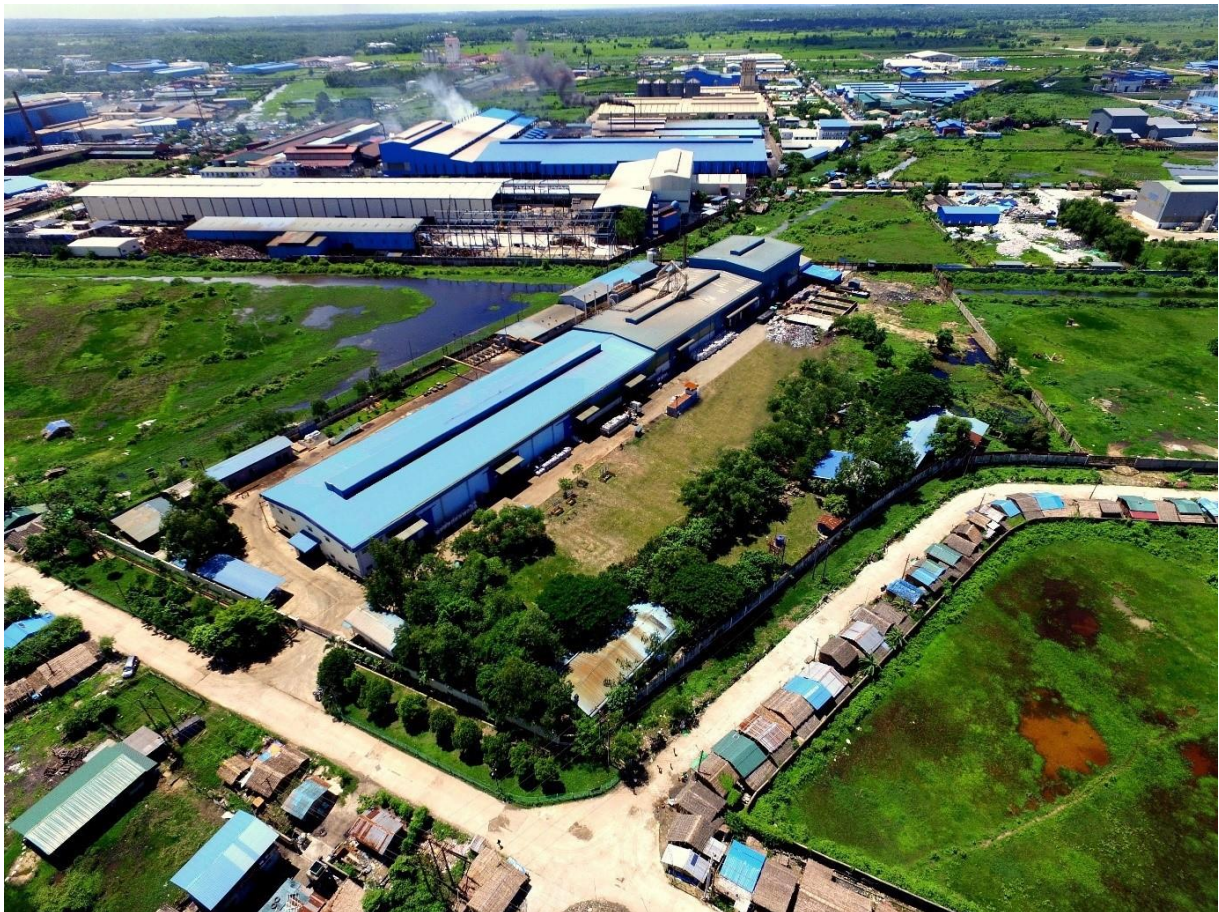
Figure 1.2-1: Factory Area and its Environments of Yangon Metal Industry Co., Ltd
