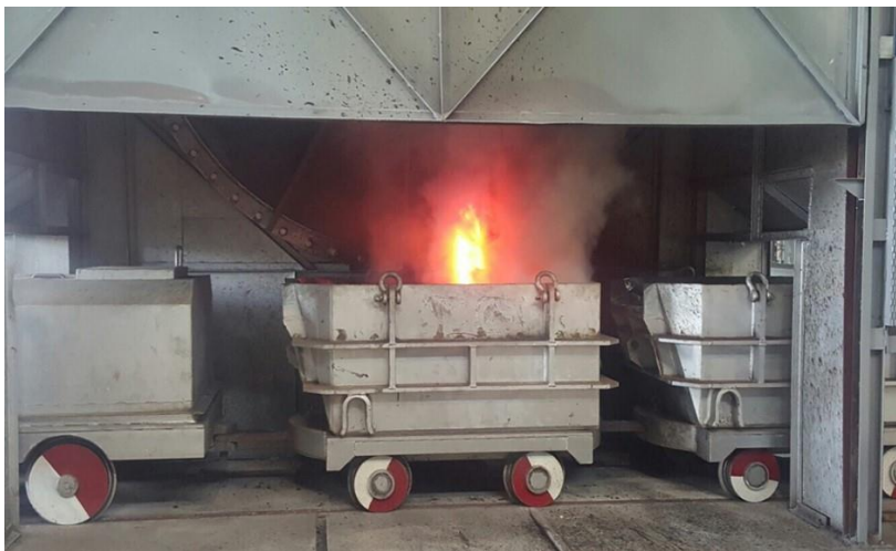
Figure 3.5-3: Rotary Smelting Furnace (Front View) (Country of Origin: Korea)
