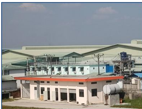
Power Station Generator Room and Fuel Storage Room
