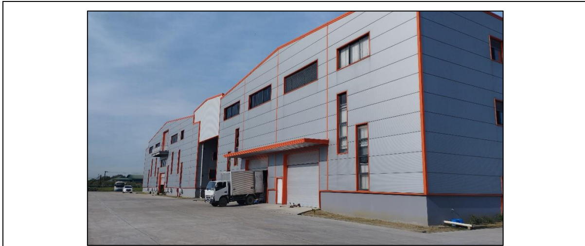
Current Construction Situation of the Project Phase 1 (Warehouse and Workshop)
