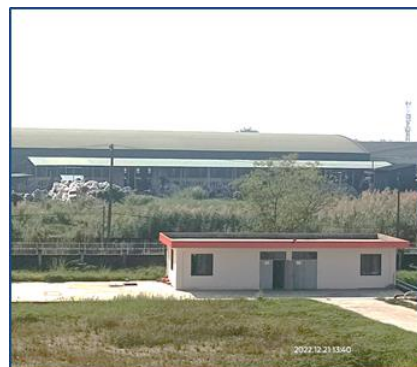
Underground Fire System Pool and Water Storage Tank
