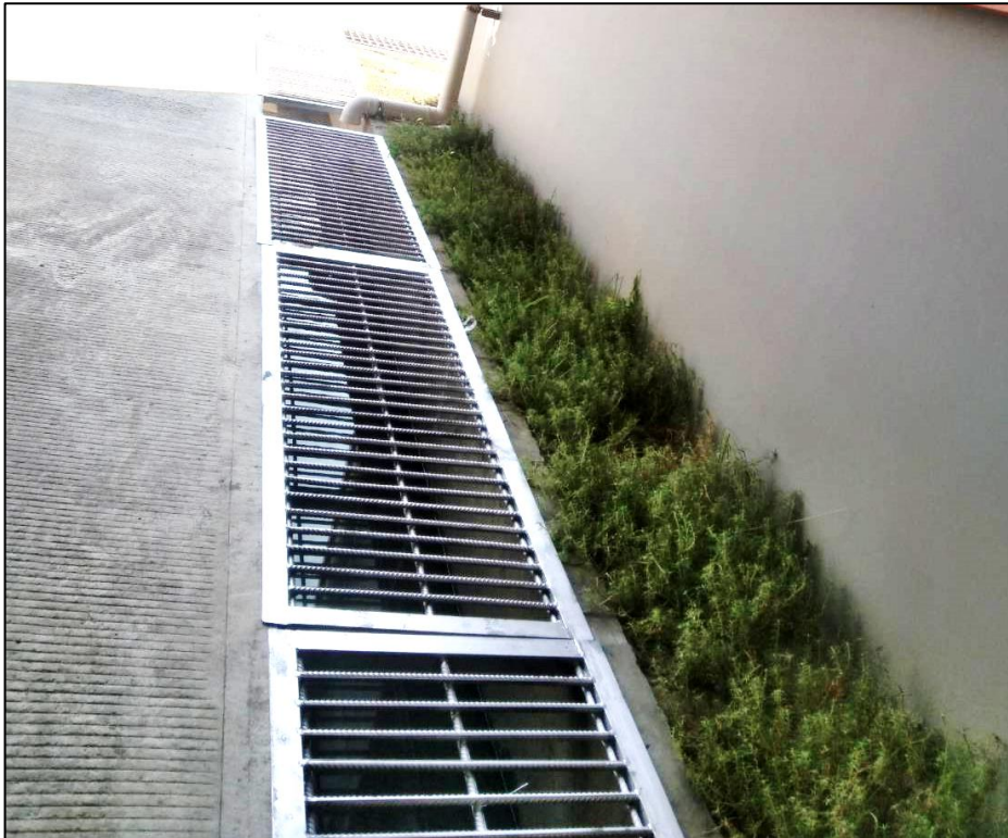
Figure 3-19 Current Situation of Drainage Channel Construction
