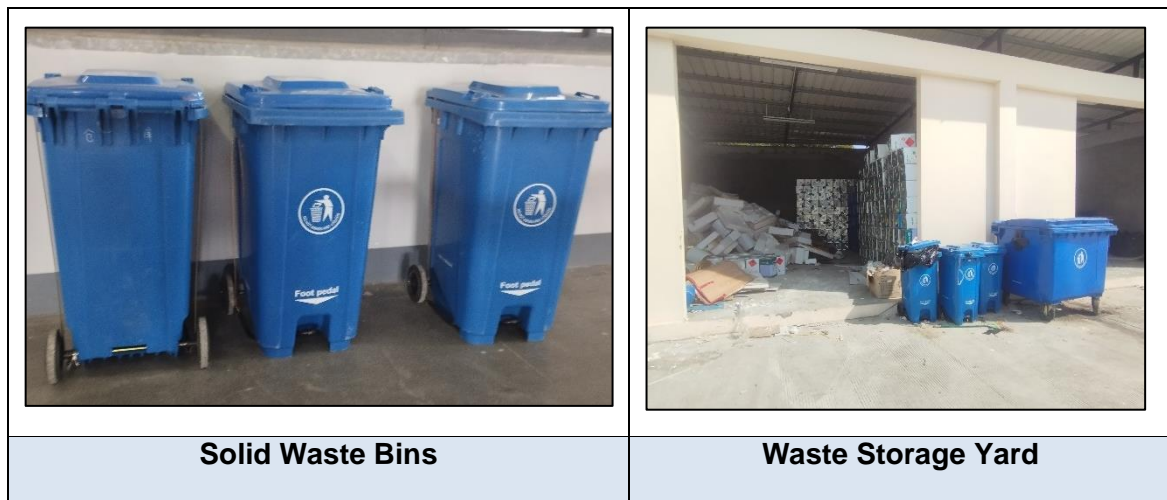
Figure 3-20 Solid Waste Bins and Waste Storage Yard
