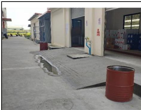
Dangerous Goods Warehouse
