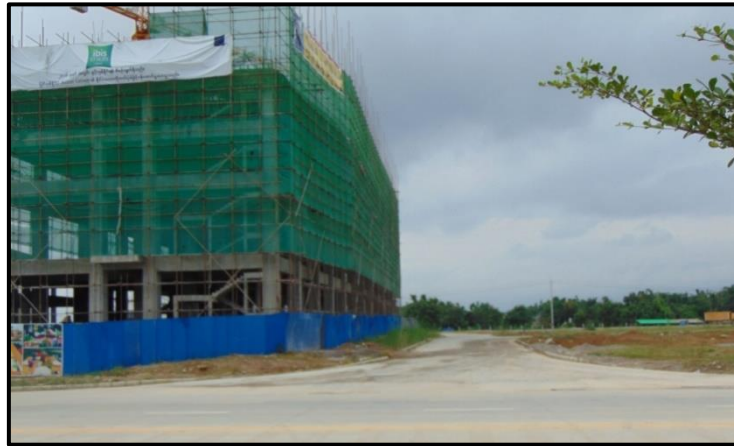
Figure 3-6 Construction in Progress (Left Sided View)
