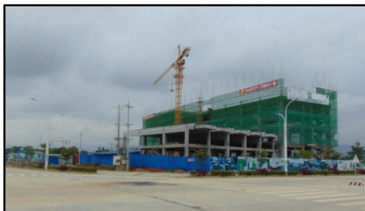
Figure 3-5 Construction in Progress (Right Sided View)
