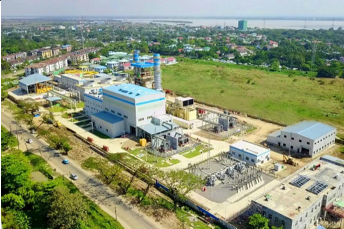
Figure 3.3-1 A Full View of the Tharketa Power Plant
