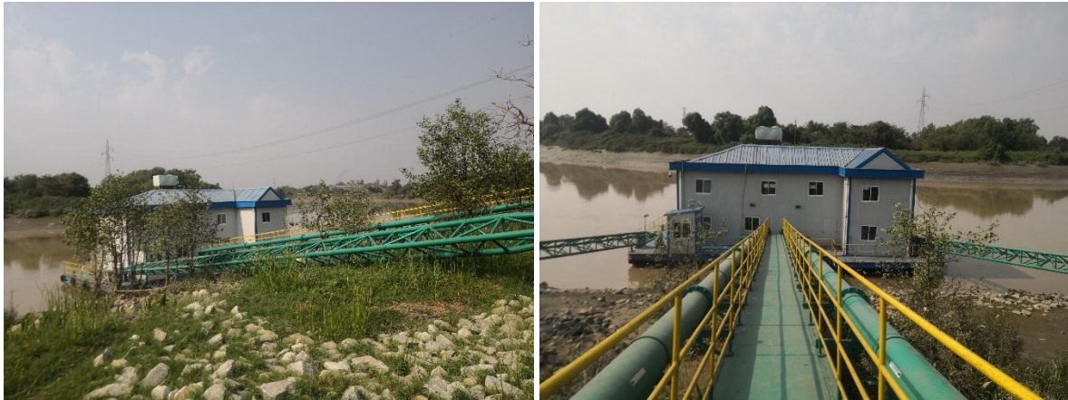
Figure 3.5-1: Floating Water Pontoon
