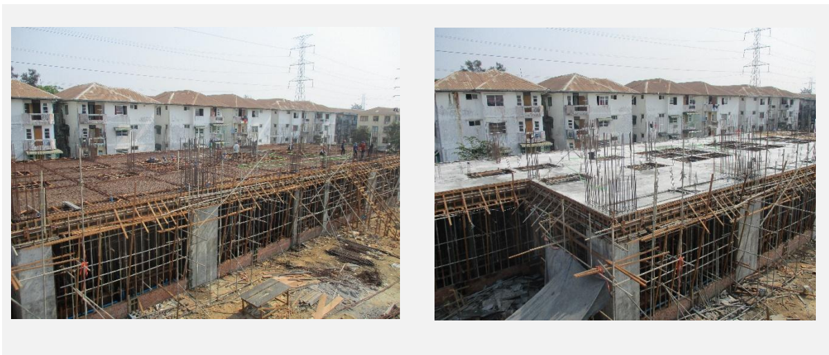
Figure 3.3-3 Construction Records of Canteen and Dormitory
