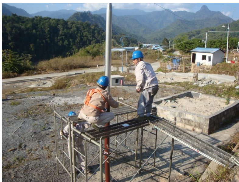
Lightning Rod for Oil Depot
