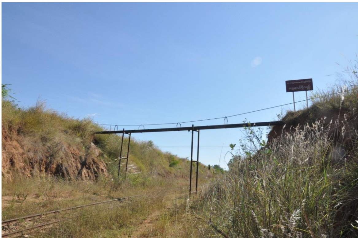
AP10 Point (N 20°10'33", E 94°51'05") Overhead Crossing
