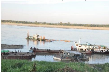
Jetty - Ayeyawaddy River
