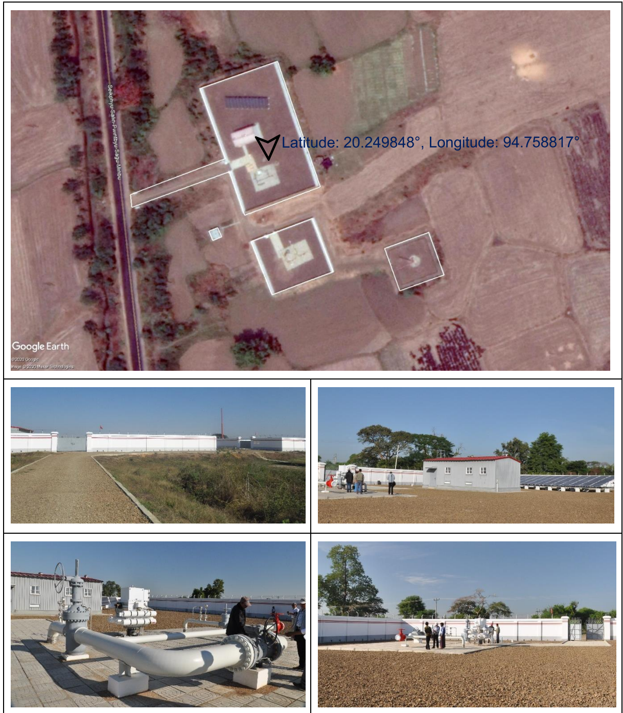
Figure 13: Off-Take Point Station
