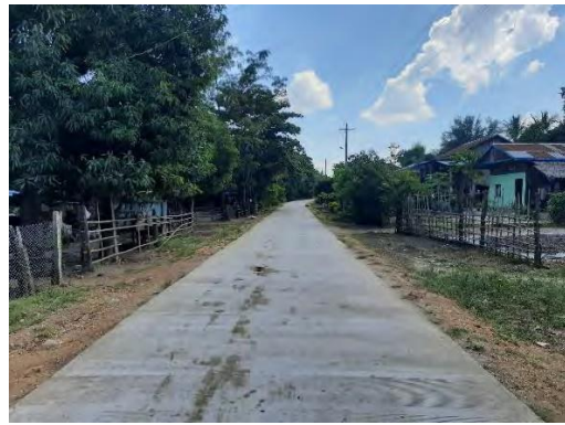
Photo Plate 5.45: Concrete Road at Myaung Shea Village
