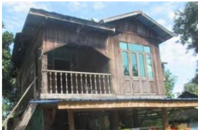
Photo Plate 5.37: Wooden Houses in the Study Area
