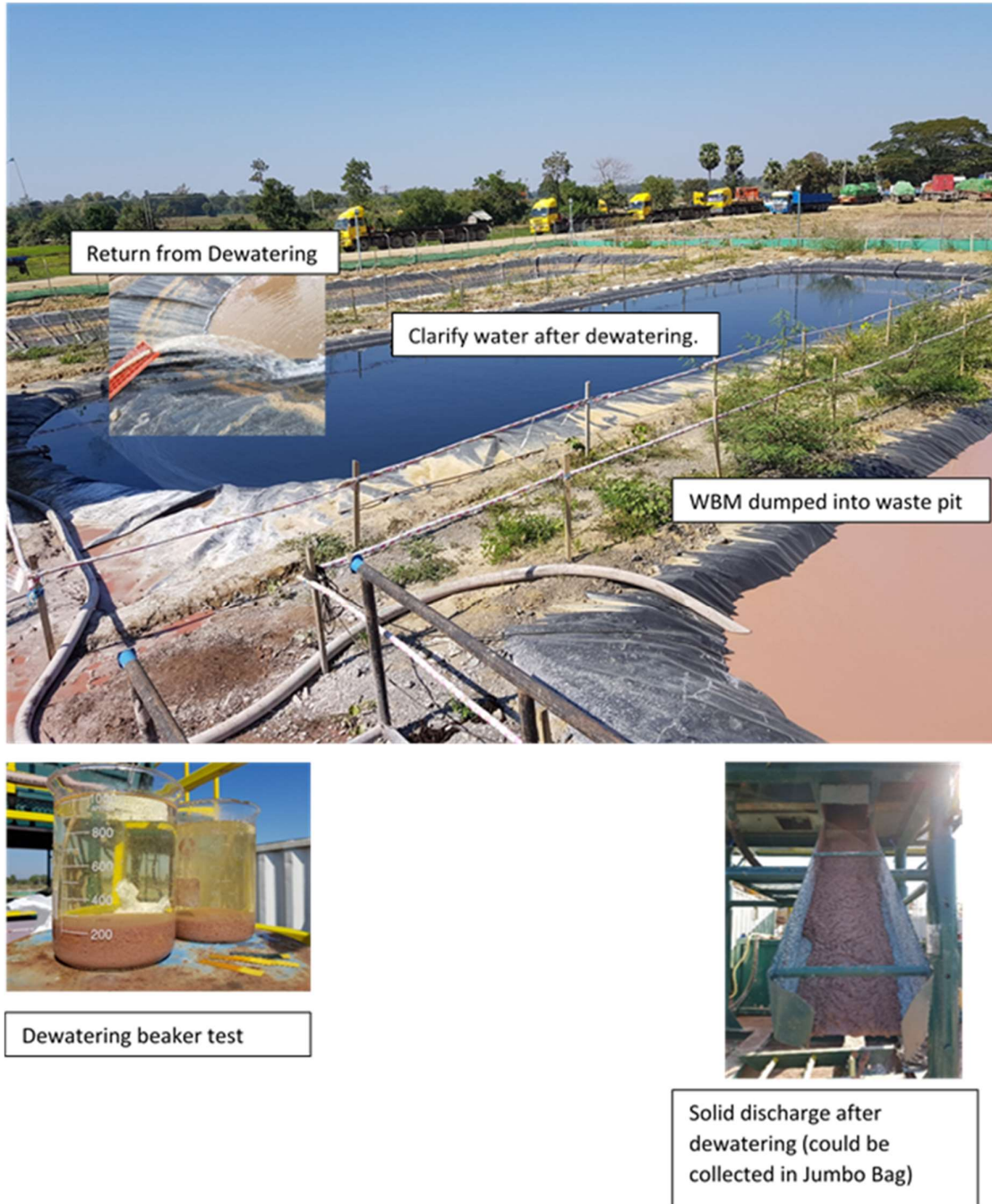
Figure 4.32: Example of Temporary Solid and Liquid Waste (1 of 2)
