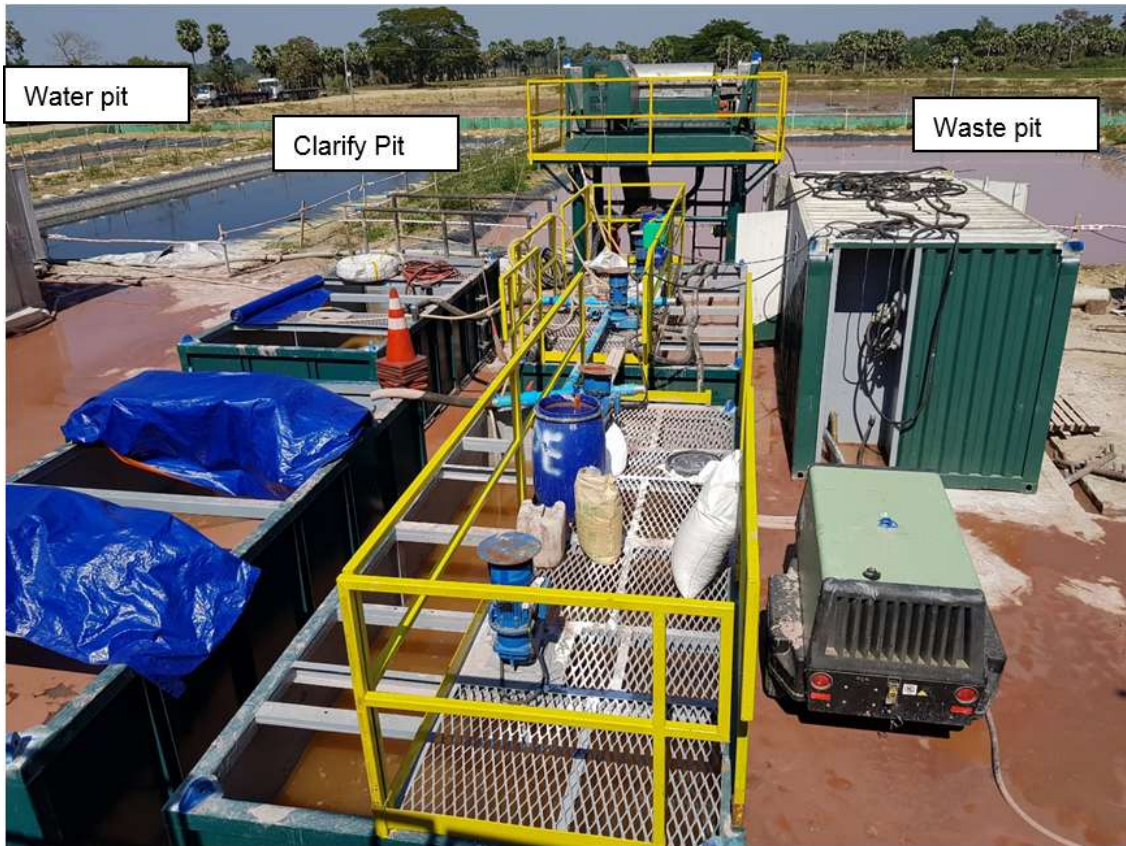
Figure 4.33: Example of Temporary Solid and Liquid Waste (2 of 2)
