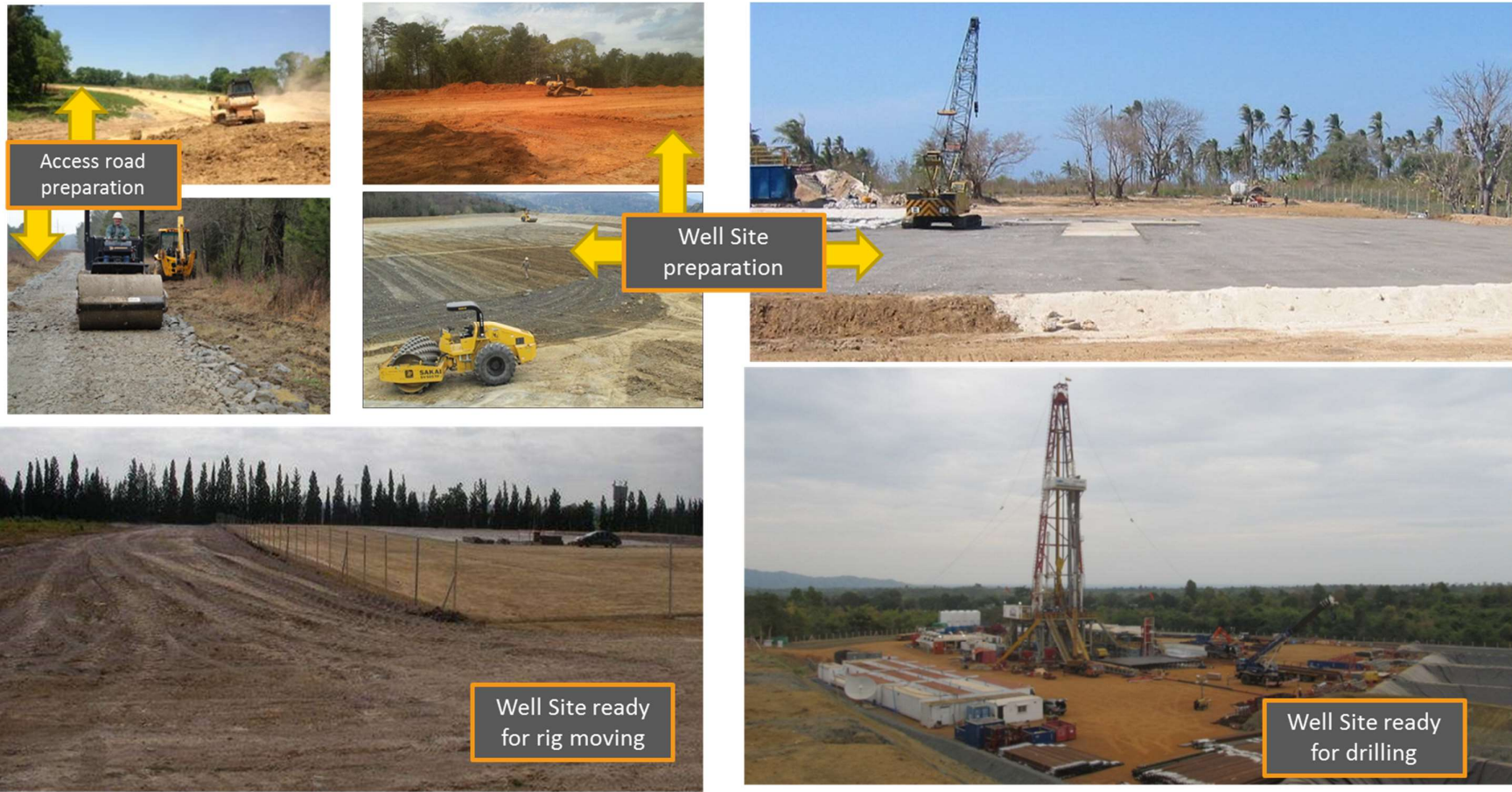
Figure 4.7: Example Images of Well Pad Construction Process
