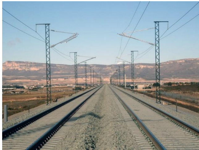
Figure - Future Railway Transmission Line
