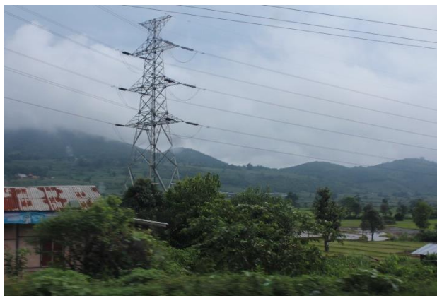
Figure - Existing Power Transmission Line in Northern Shan Region
