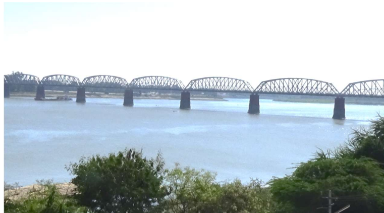
Figure - Innwa Bridge
