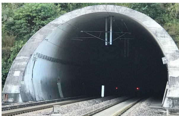
Figure - Drop tube suspension for double-track tunnel
