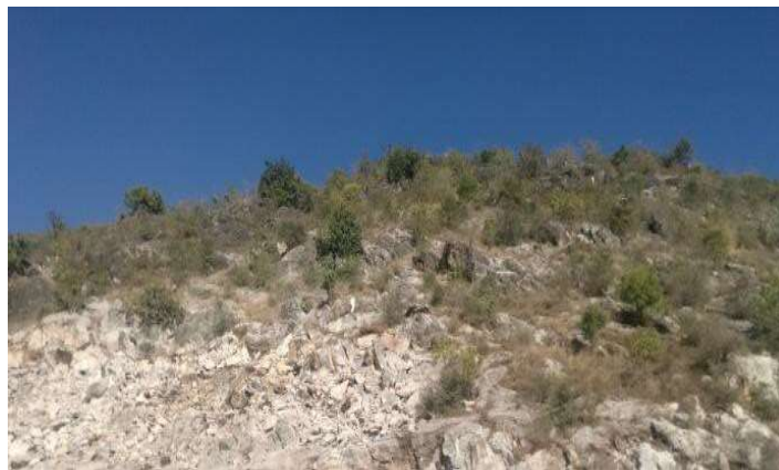
Dangerous Rock and Rockfall
