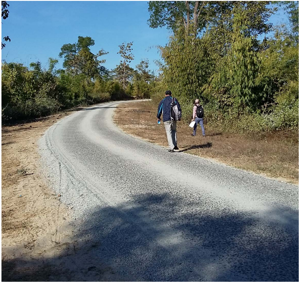
Figure 4.5 Photos showing Condition of Existing Access Road in PSC H
