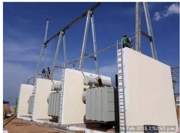
**Figure 4-11: Main Transformer Installation Work**
