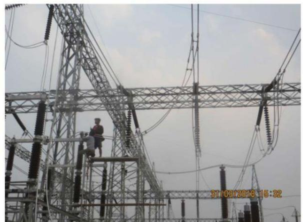
**Figure 4-12: Bus Installation Work**
