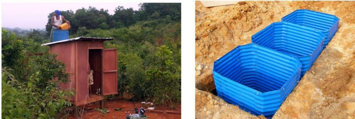
**Figure 4-20: Septic tank, aerobic tank and sedimentation tank and Toilet**
