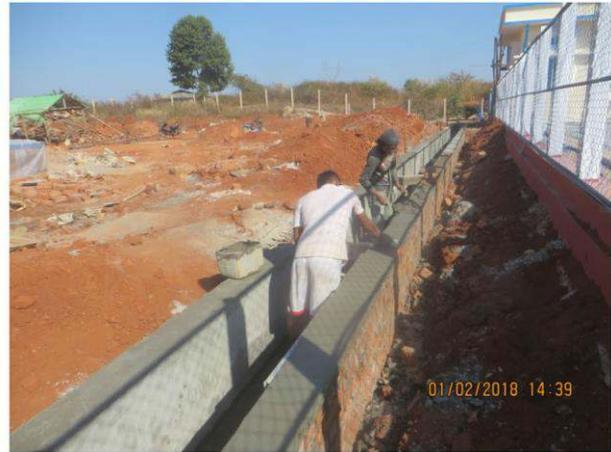
**Figure 4-8: Switchyard Drain Work**
