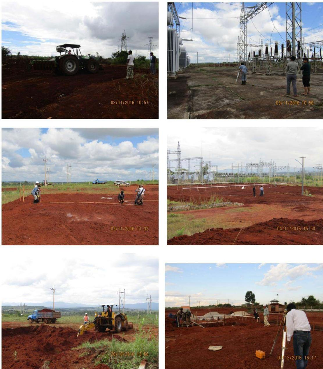
**Figure 4-5: Site Survey, Site Cleaning & Cutting & Filling Work**
