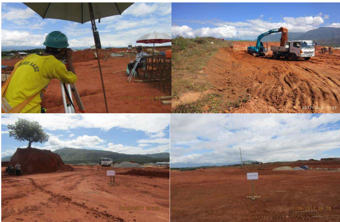
Figure 4-3 Site Survey, Site Cleaning & Cutting & Filling Work
