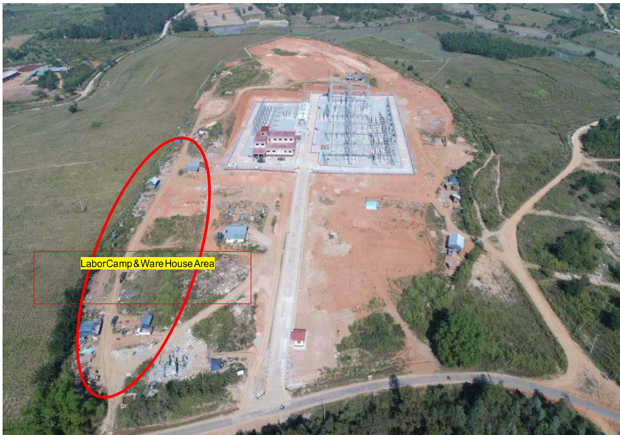
Figure 4-19 Labour House and Warehouse area
