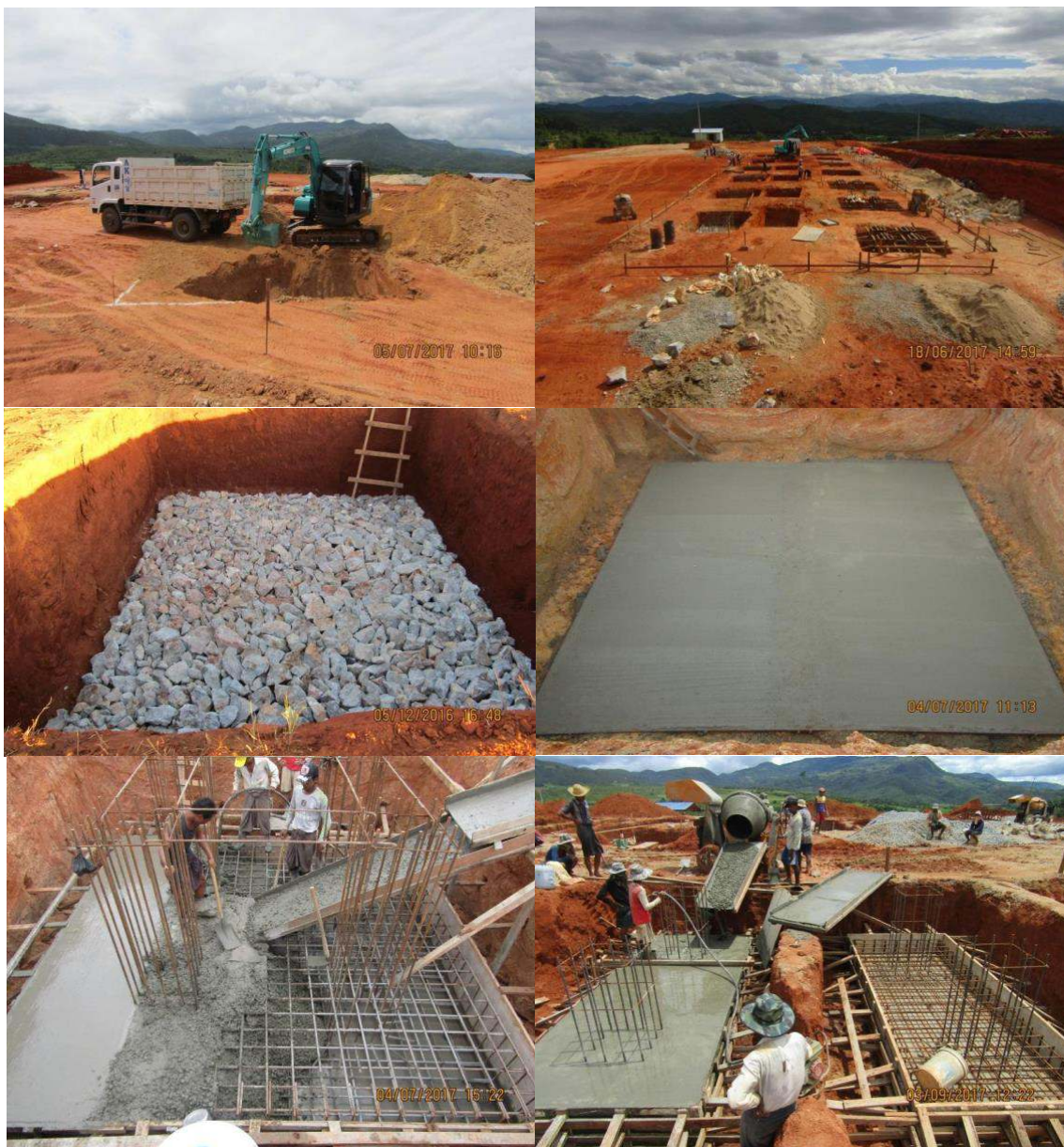
Figure 4-4 Foundation Work (Excavation, Hardcore Filling, Lean Concrete, Rebar Install, Concrete Work)
