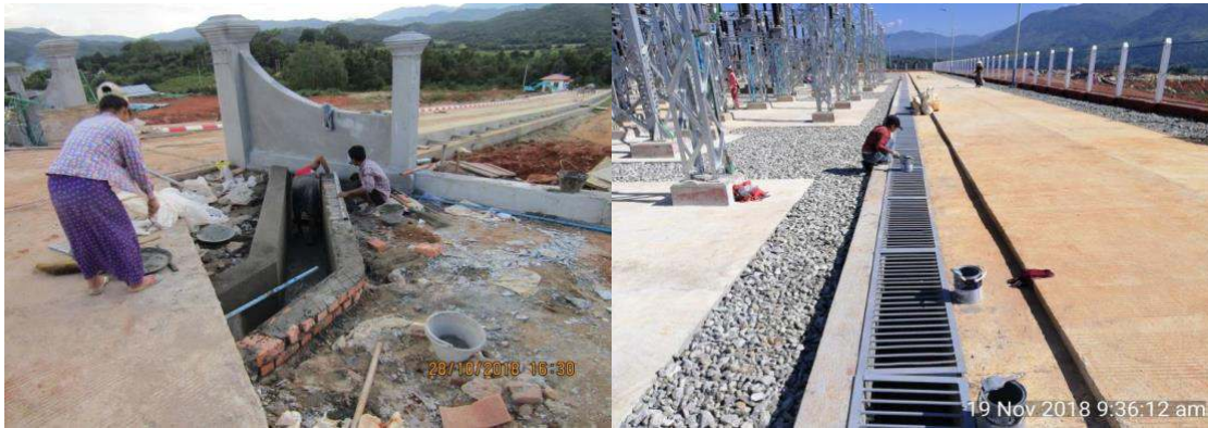
Figure 4-7 Switchyard Drain Work
