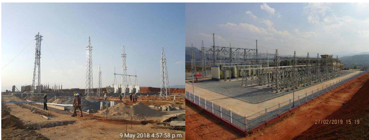
Figure 4-9 Structure Erection Work
