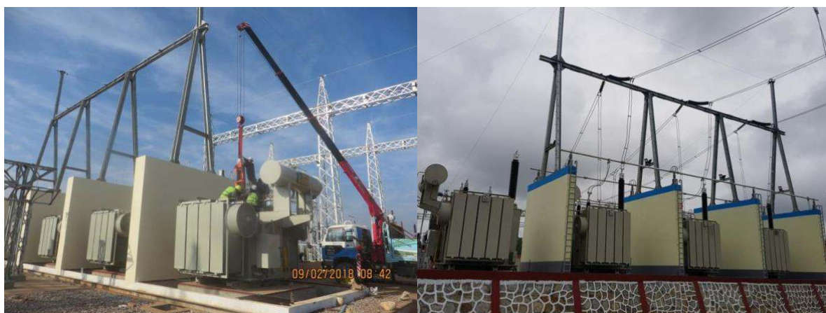
Figure 4-11 Main Transformer Installation Work
