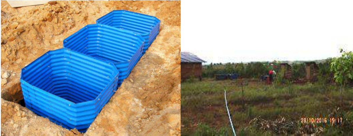
Figure 4-20 Septic tank, aerobic tank and sedimentation tank and Toilet
