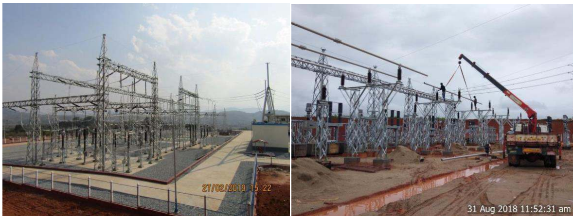
Figure 4-12 Bus Installation Work
