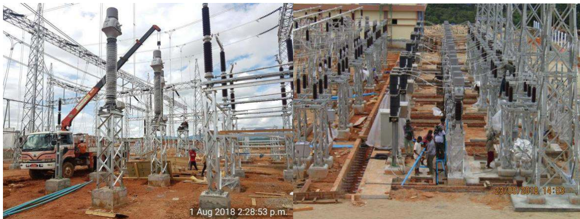
Figure 4-10 Equipment Installation Work
