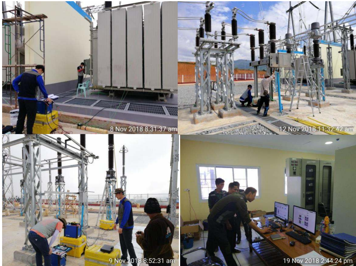
Figure 4-14 Testing & Commissioning Work
