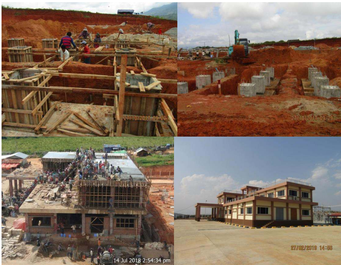
Figure 4-5 Control Building Work
