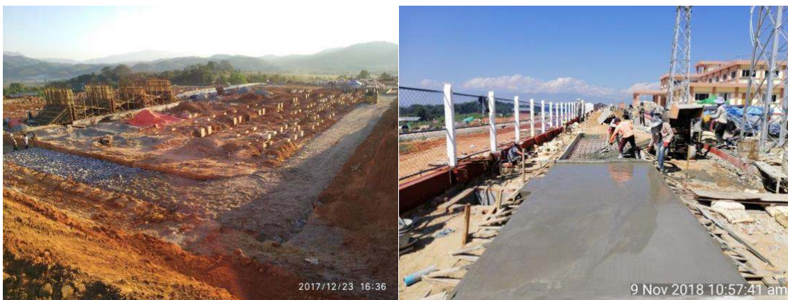
Figure 4-6 Access Road Work
