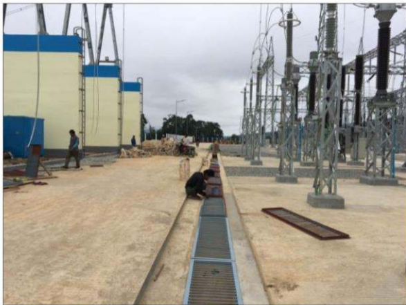
Figure 4-10: Switchyard Drain Work
