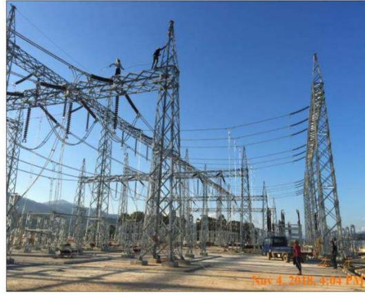
Figure 4-14: Bus Installation Work
