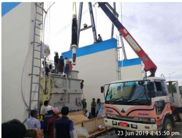
Figure 4-13: Main Transformer Installation Work
