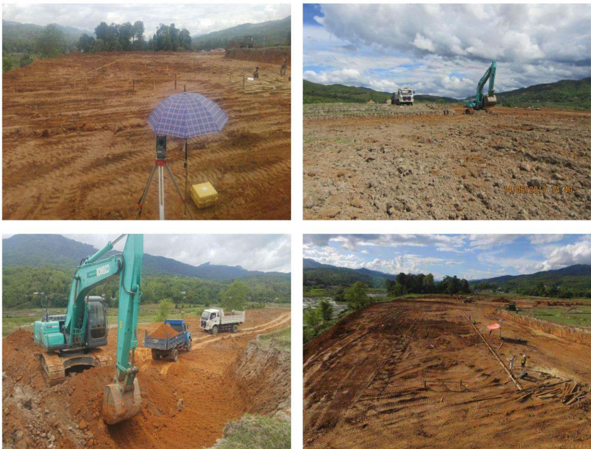
Figure 4-5: Site Survey, Site Cleaning & Cutting & Filling Work
