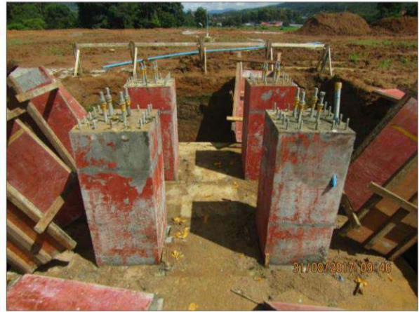
Figure 4-6: Foundation Work (Excavation, Hardcore Filling, Lean Concrete, Rebar Install, and Concrete Work)
