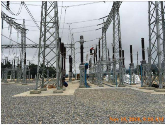
Figure 4-14: Bus Installation Work
